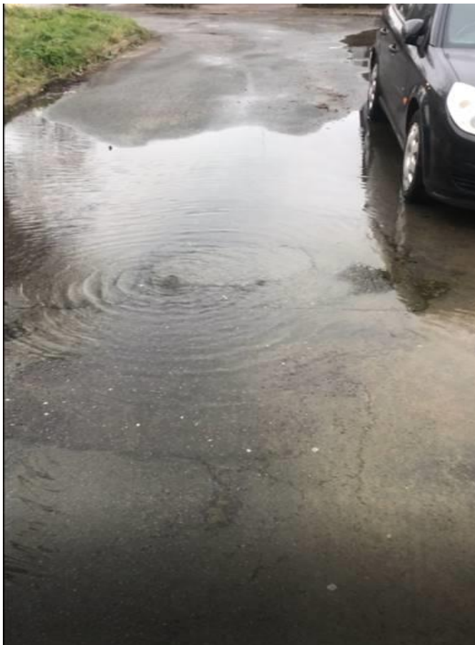
Groundwater emergence in mini crescent for 68 – 78 Old Shoreham Road.
