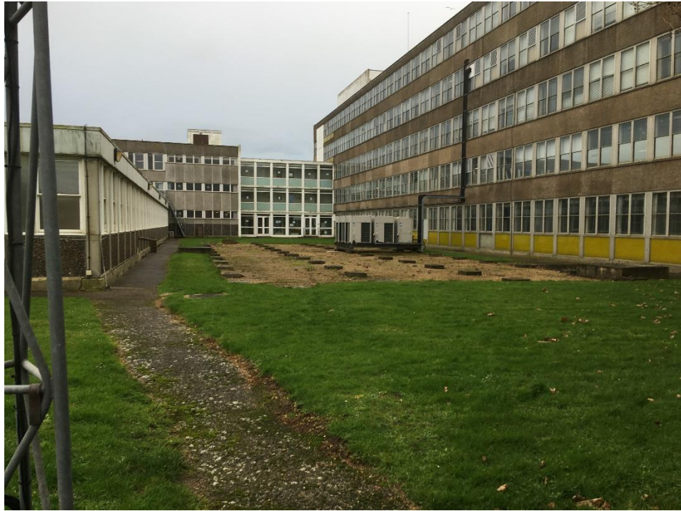
Photograph 04 - View of part of the main complex to the north of the site. View looking south
