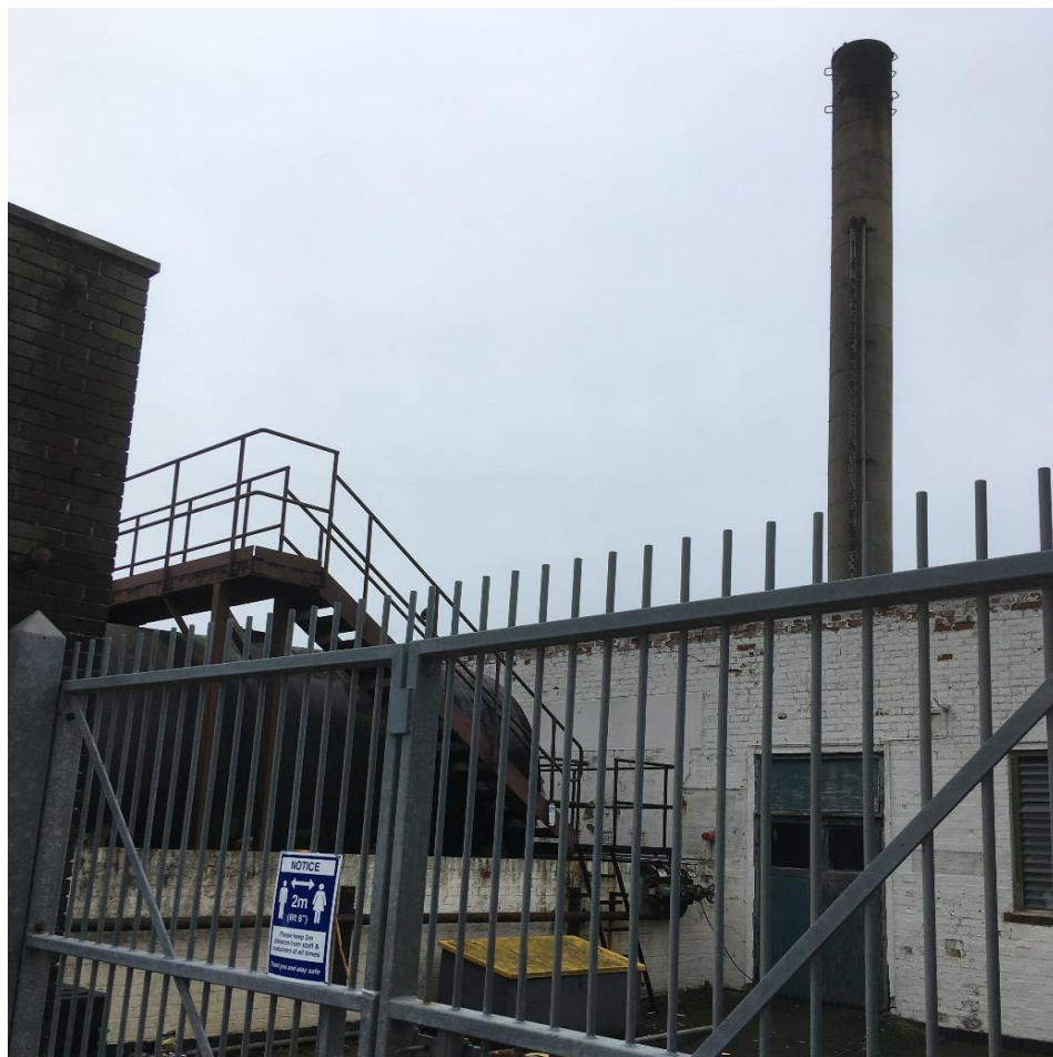
Photograph 03- View of the maintenance area showing oil tank, typical building and chimney on site. View looking north-west.
