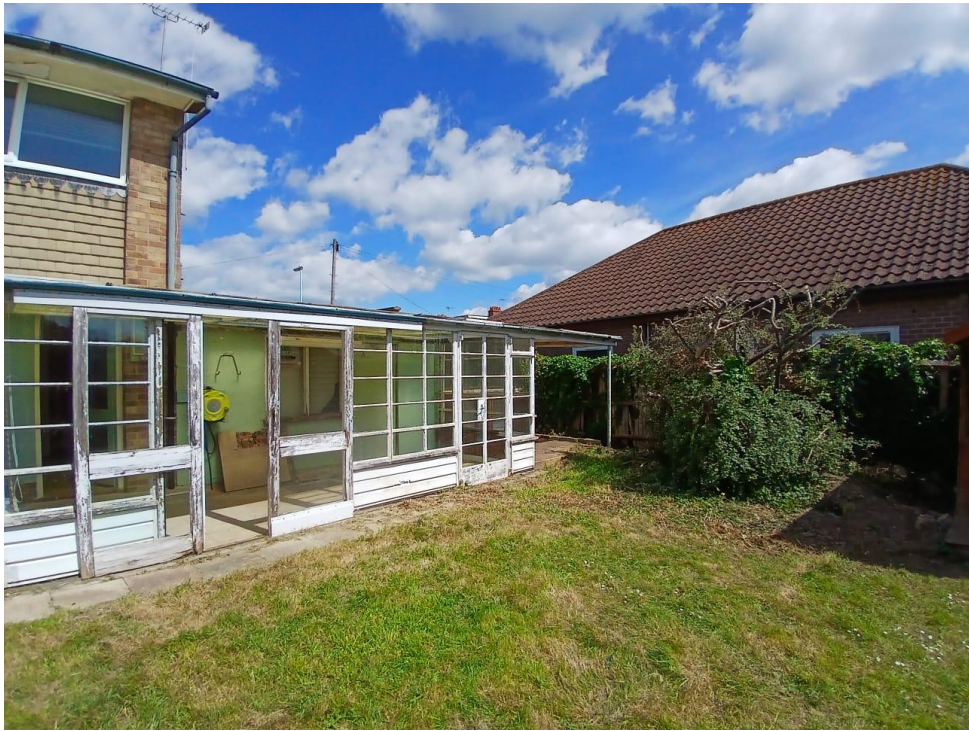
Photograph No. 2: Rear garden of existing residential building
