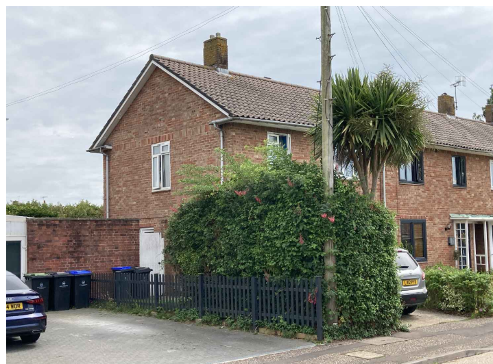
Photo 3: Existing side elevation
