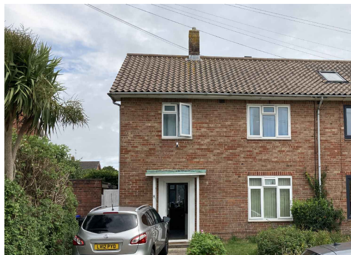
Photo 1: Existing front elevation
