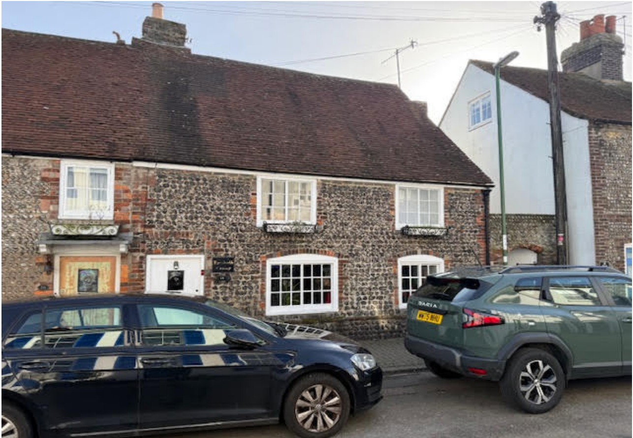
Fig.1 - Front Elevation of 14 West Street. (White door main entrance).
