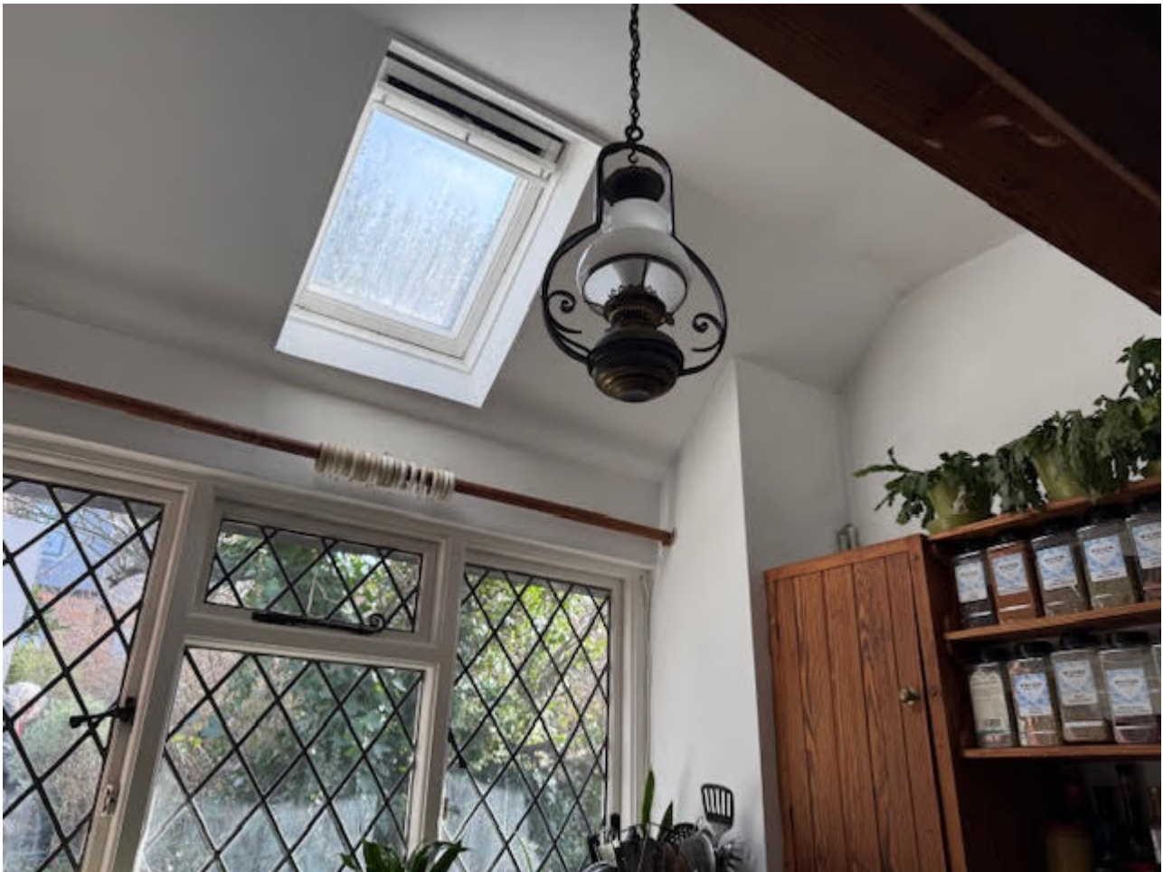
Fig. 6 Existing part vaulted ceiling to Kitchen with rooflight. To be replaced with more conservation style rooflight.
