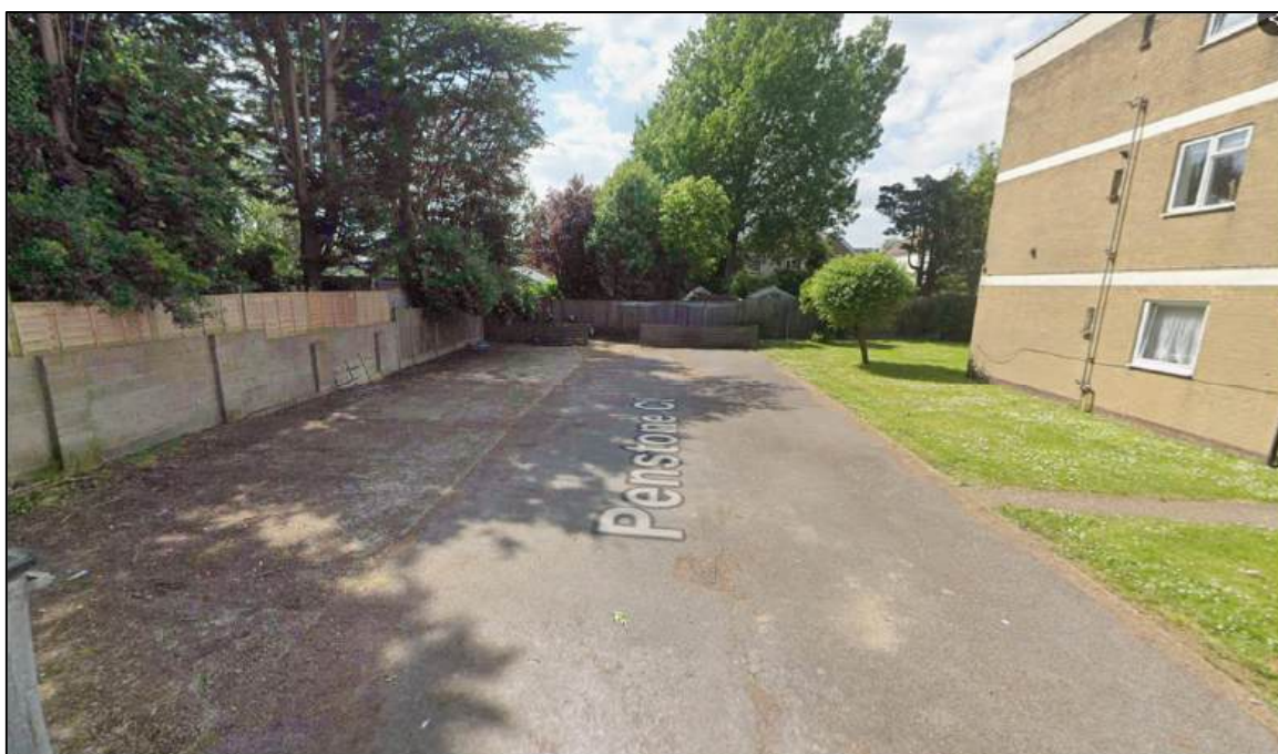
Figure 2.1 – Existing hardstanding areas to be removed
