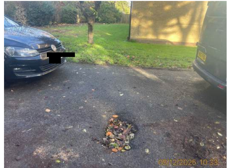
Plate 8 – drain system on southern edge by garages
