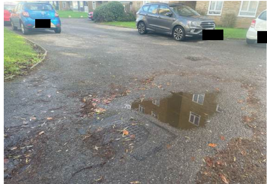
Plate 12 - continuation of water line
