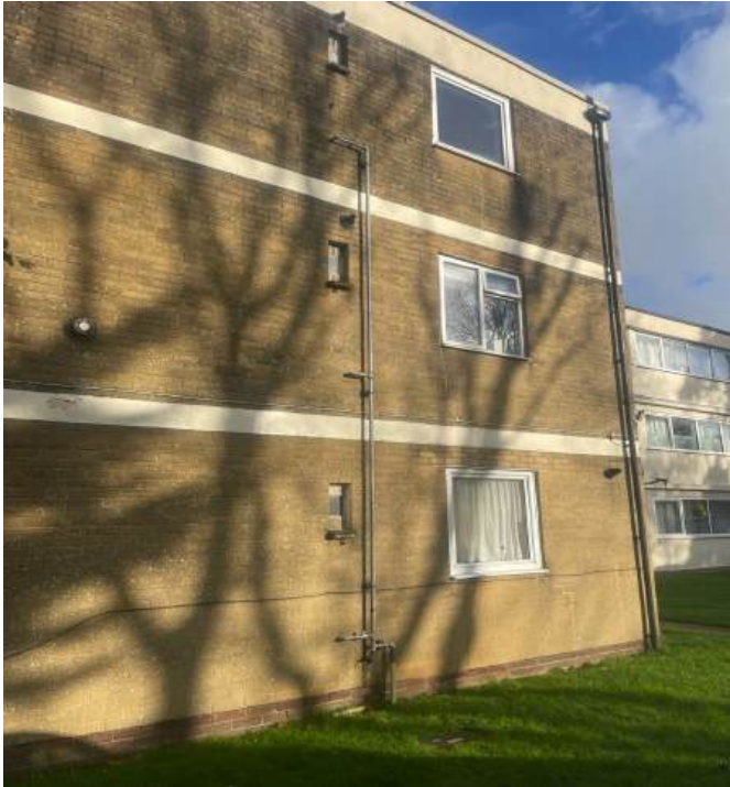
Plate 9 – Gas main down western block of flats - south side.
