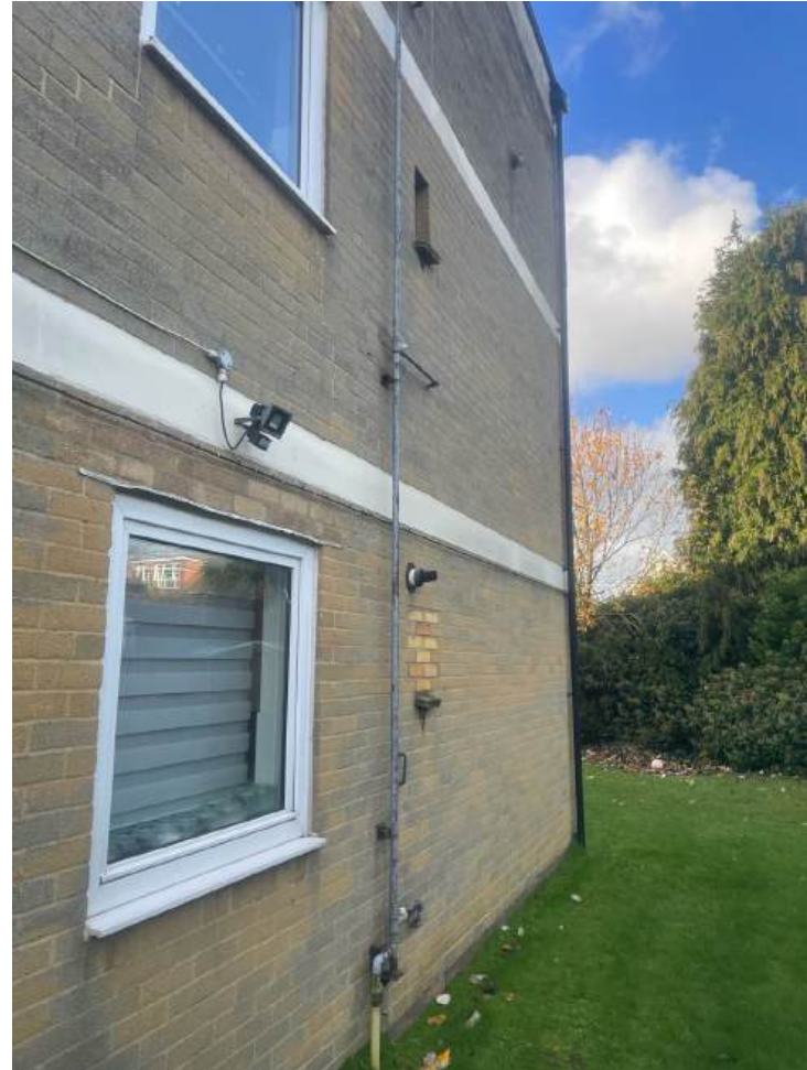
Plate 18 - gas main down northern side of site
