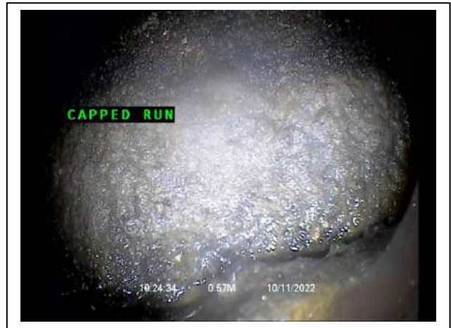
Manhole 4 – Upstream - Capped End
