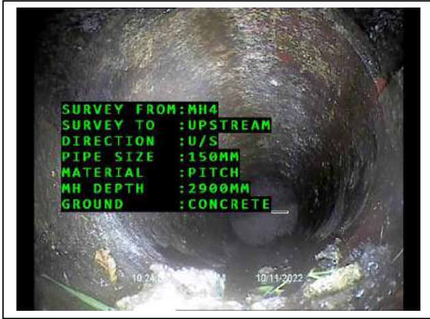
Manhole 4 – Upstream - Capped End
