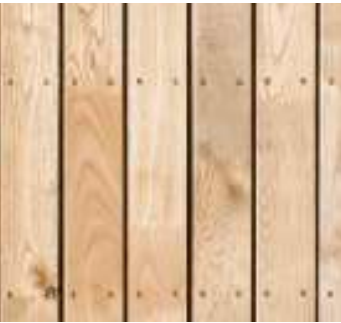
Vertical natural timber cladding
