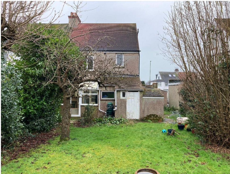
Image 03 – Rear elevation of 310 Upper Shoreham Road taken from its rear garden.
