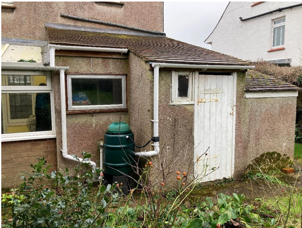
Image 05 – Single storey original elements consisting of Kitchen, WC (disused) and external store proposed to be removed.
