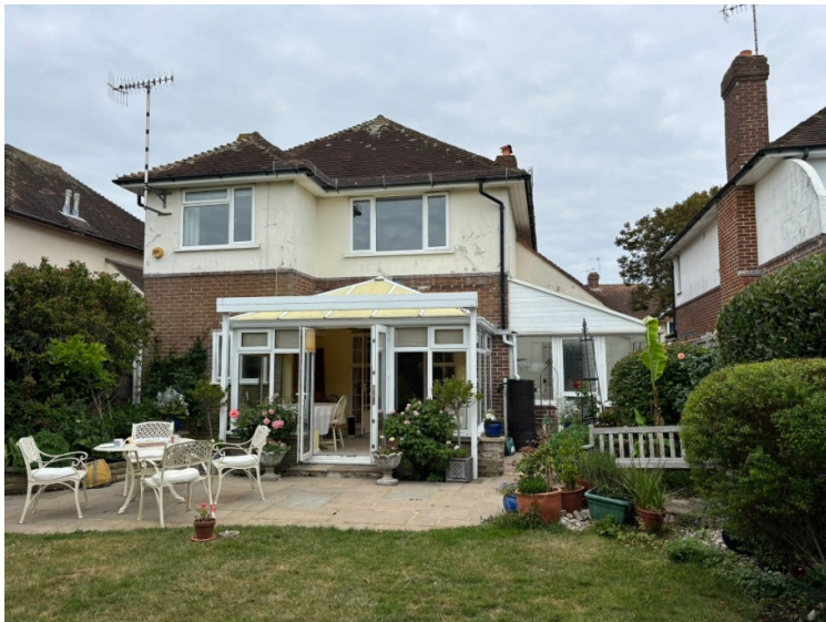
Existing rear elevation from garden
