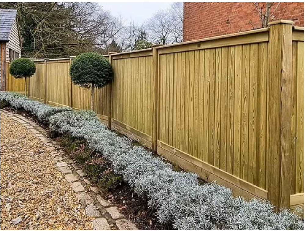
PROPOSED SOLID TIMBER VERTICAL BOARDED TONGUE AND GROOVE FENCING AND SIDE GATES
