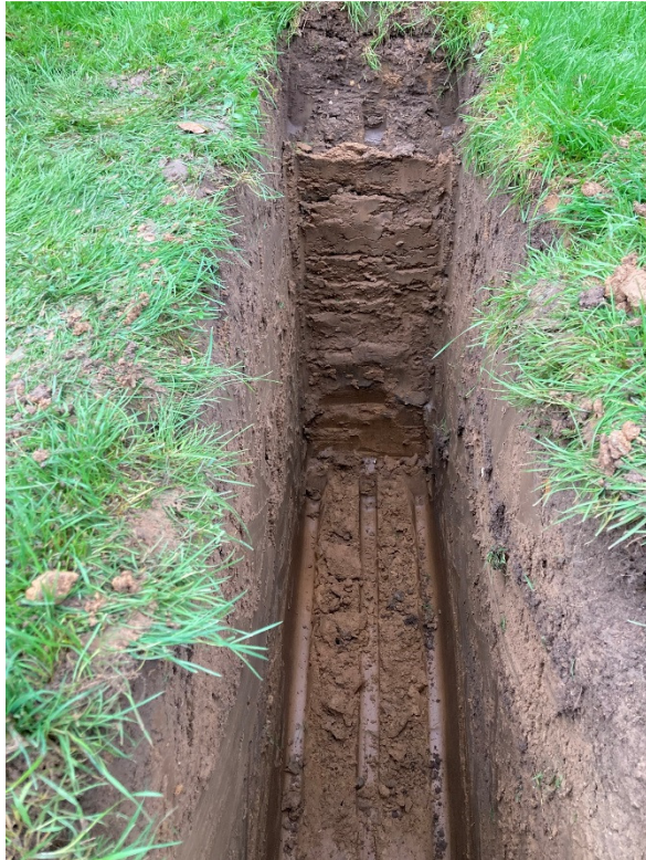
Photograph 9 : Trial Pit TP2 Excavation
