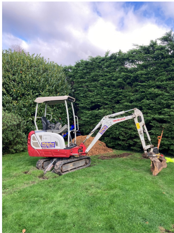
Photograph 5 : Trial Pit TP1 Location
