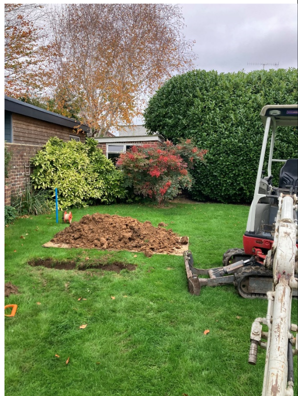
Photograph 8 : Trial Pit TP2 Location
