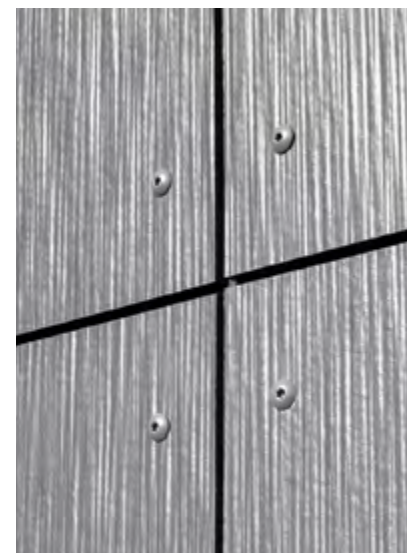
Hardie® Panel Screw Fixing
