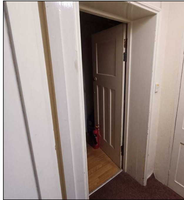
Door BD02 Basement Floor
