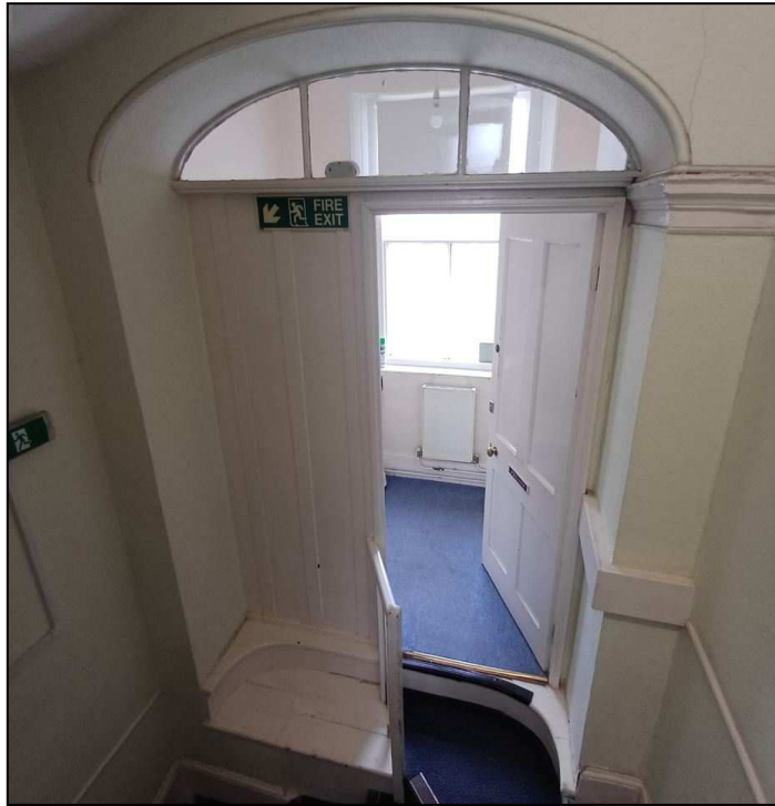
Door FD01 Intermediate landing between Ground and First Floor
