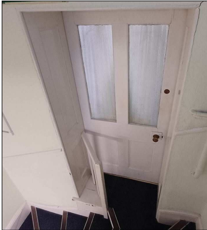
Door SD01 Intermediate landing between First and Second Floor
