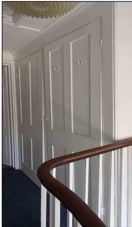
Cupboard doors TD01a and TD01b Third Floor
