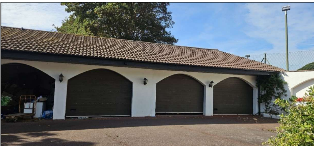
Photo 3 – The detached triple garage building, with hipped tile roof and closed eaves.
