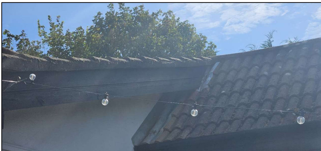
Photo 4 – Junction of two pitched roof sections in the area of the proposed works, showing closed eaves and no evidence of gaps.
