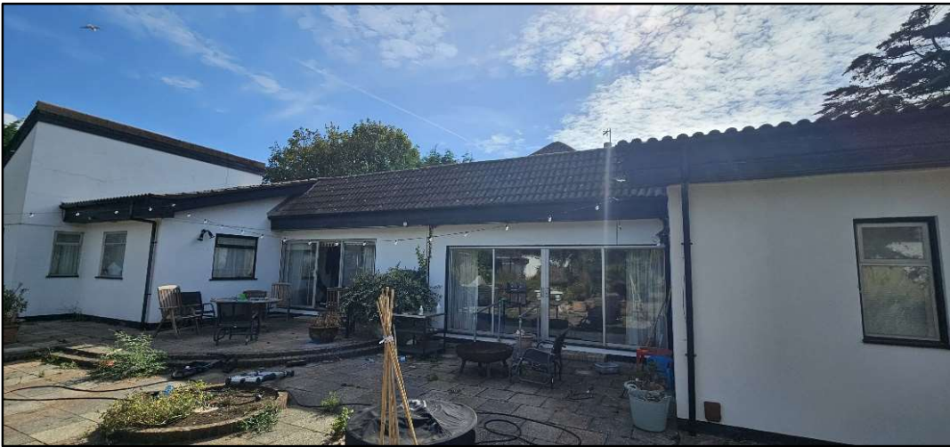
Photo 2 – Photo showing photovoltaic (PV) panel installation to the rear roof slope.
