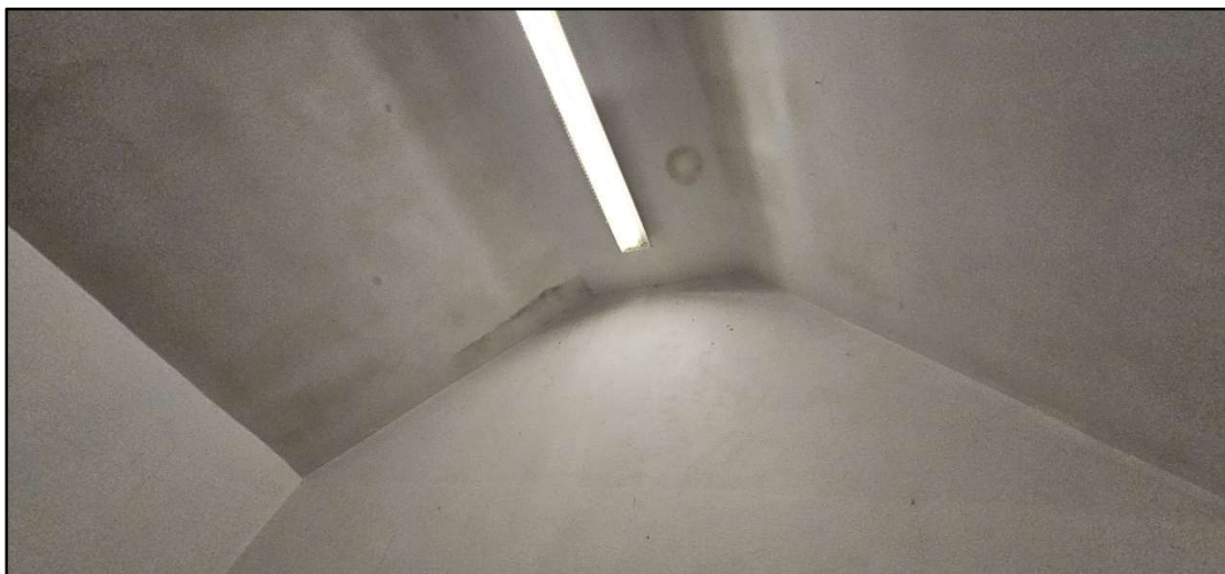
Photo 5 – Interior of the existing loft spaces, in the areas of the proposed works.
