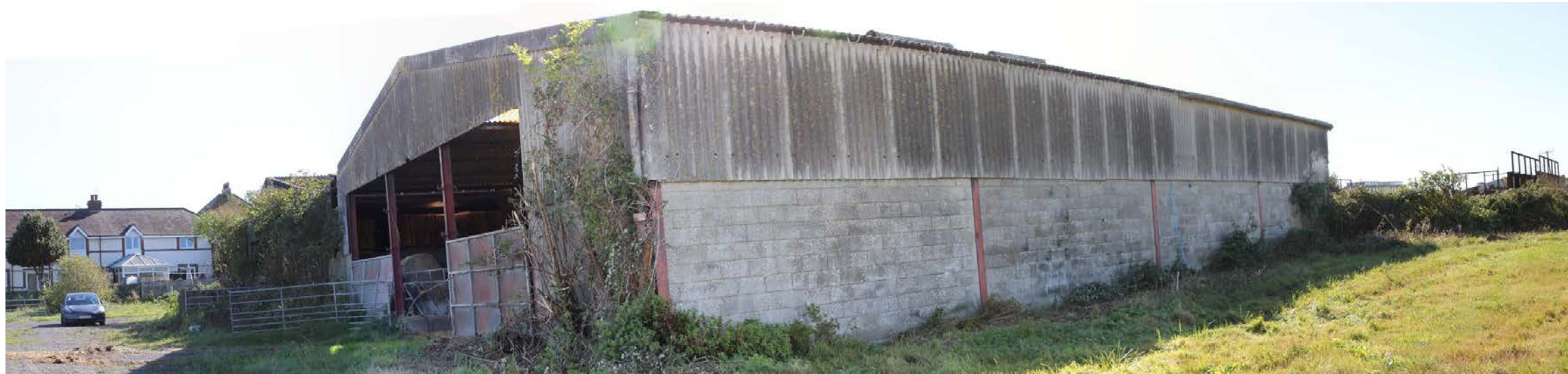
Photograph B - From the northwestern corner of the Site
