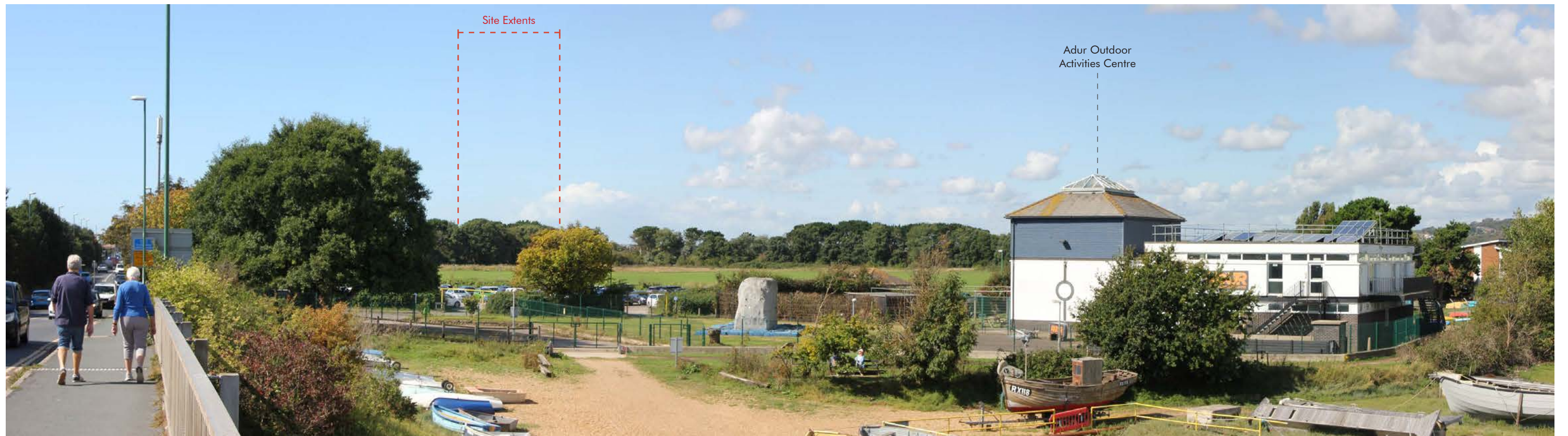
View 6 - View looking west from the Norfolk Bridge as it crosses the River Adur, adjacent to the Adur Outdoor Activities Centre
