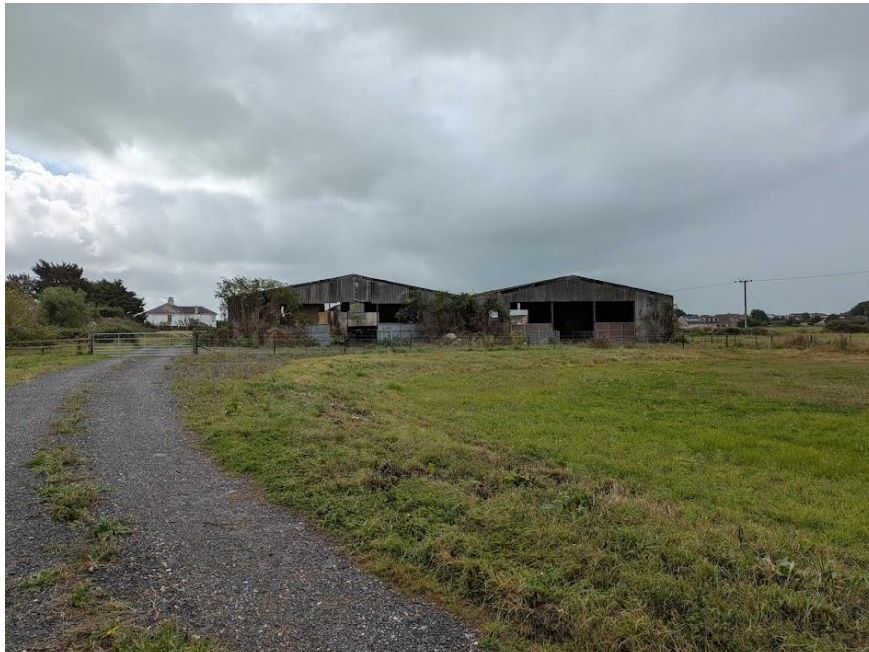
Photo 5. View of the Site facing southwards.
