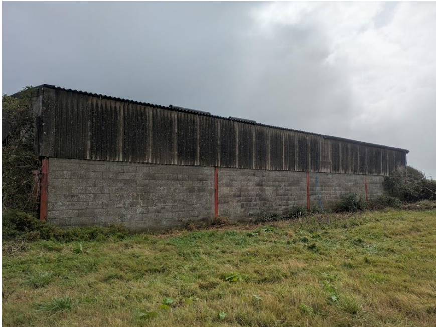
Photo 11. Western side of adjoining barns.
