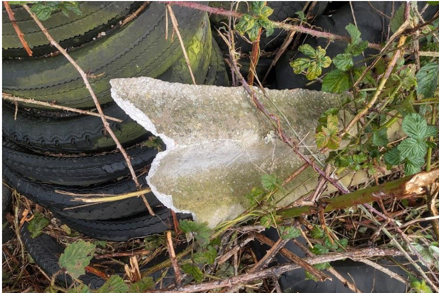
Photo 21. Cement sheeting fragment observed to the south of the southern barn.
