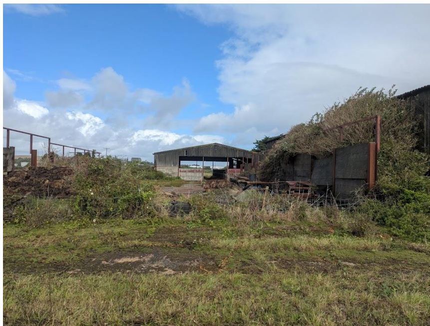
Photo 22. Former barn structure in the south-west of the Site (looking northwards).
