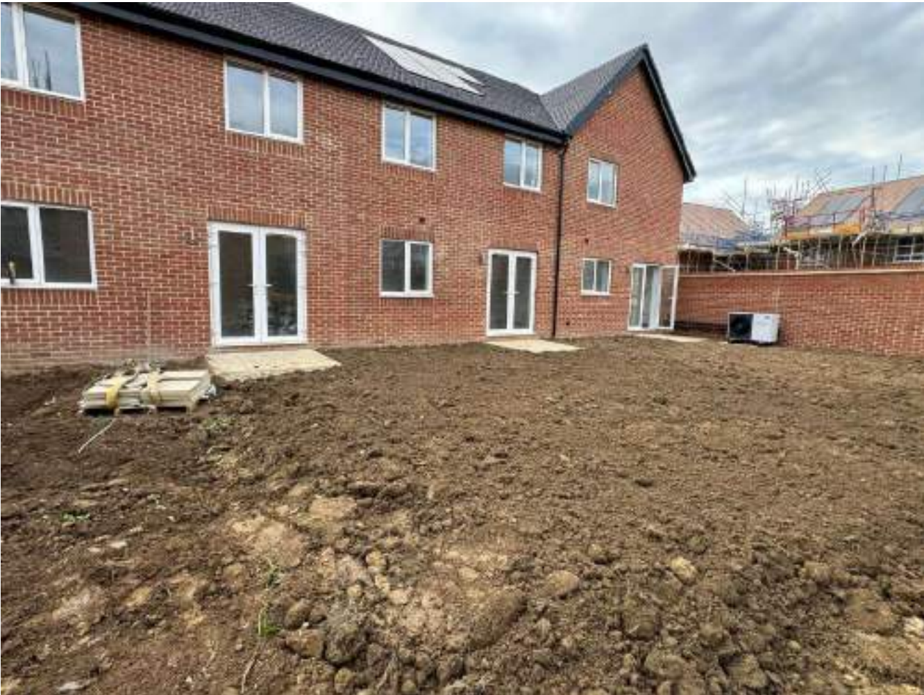
Plots 107 – 109: contractor supplied photo following placement of topsoil. Dates 24.09.2025
