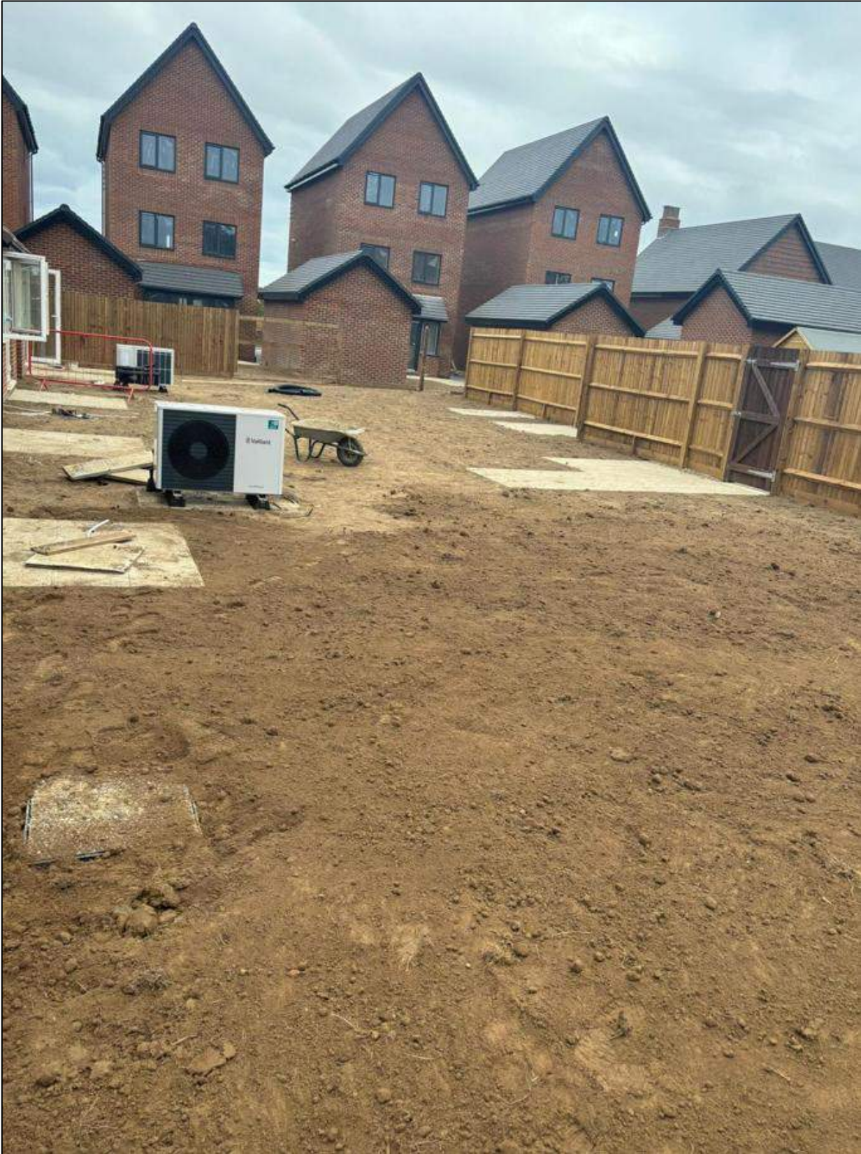
Contractor photograph following completion. Plots 130 – 133
