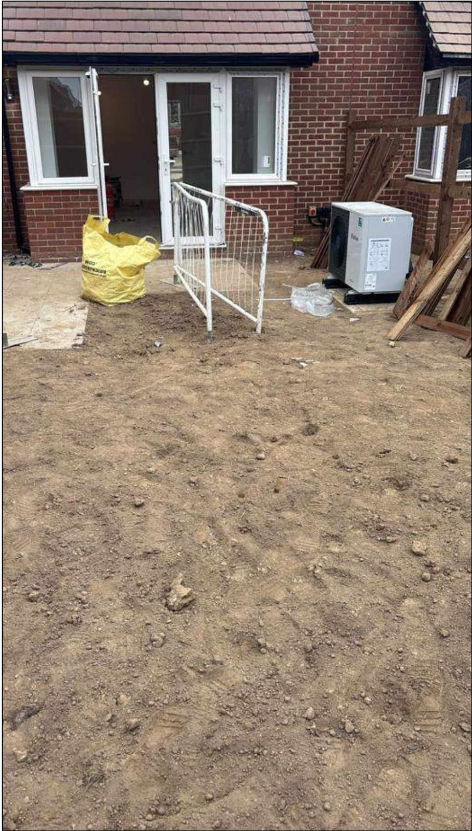
Contractor photograph following completion. Plots 139
