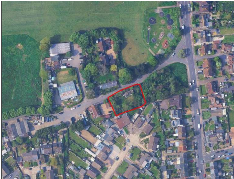
Figure 3-1 Site location and the surrounding area (evidence of fire damage to the existing Thatch Cottage building can also be seen)
