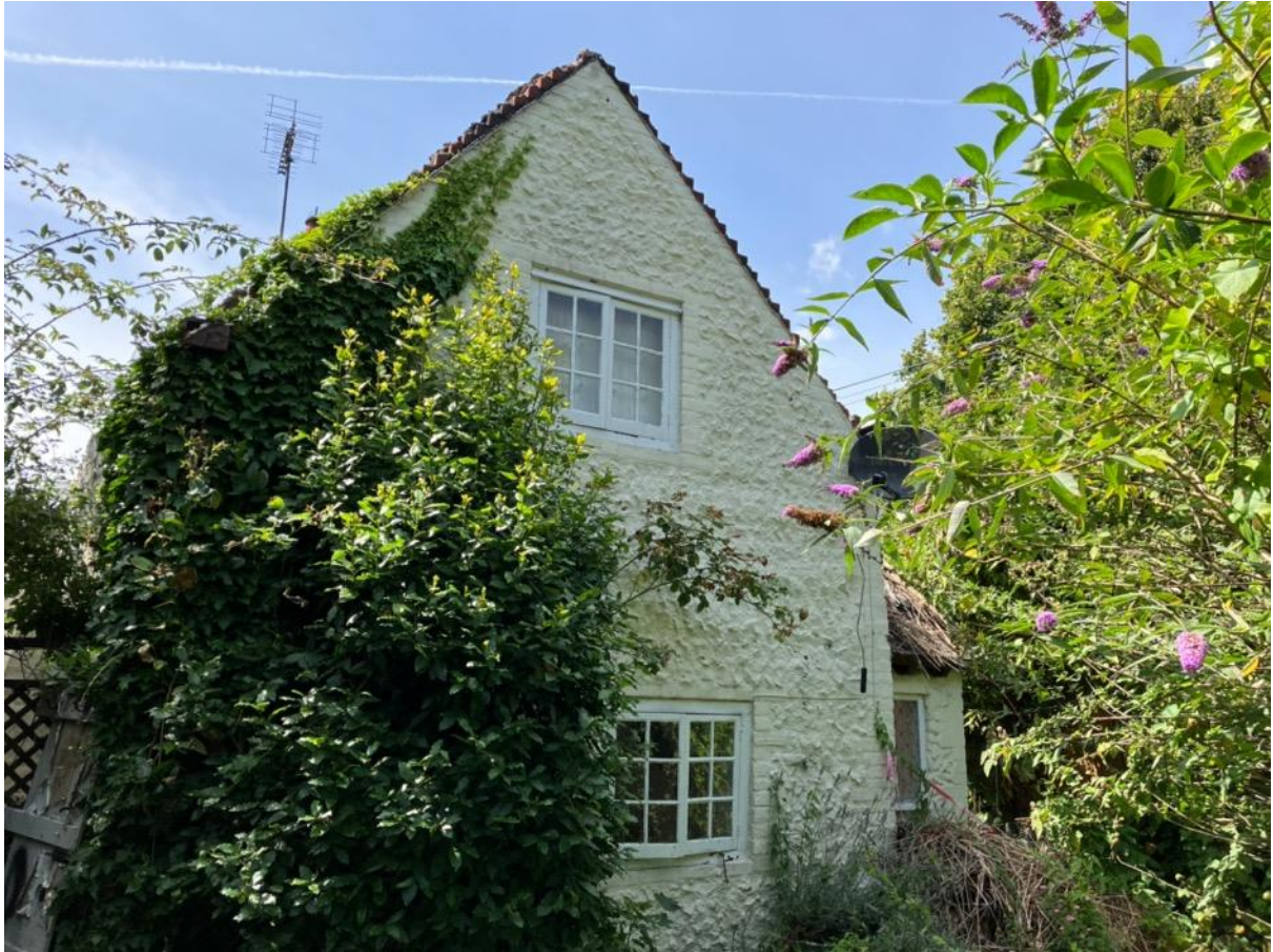
Photograph 3. The eastern aspect of the property as taken in July 2023.
