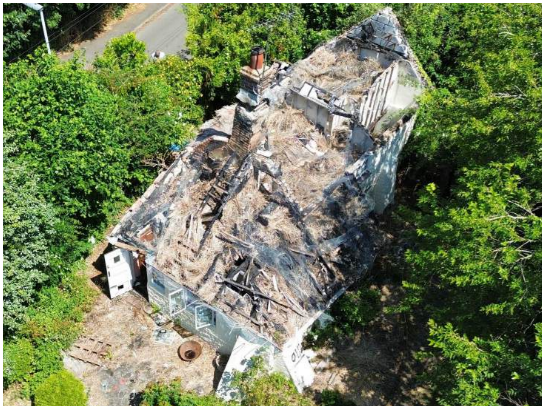
Aerial view from the west, summer 2023.
