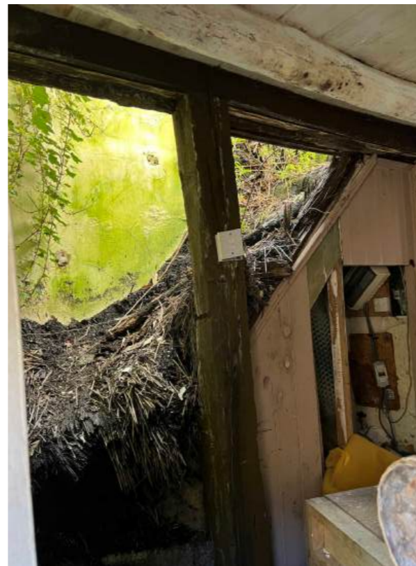
Stairwell looking south, spring 2025.
