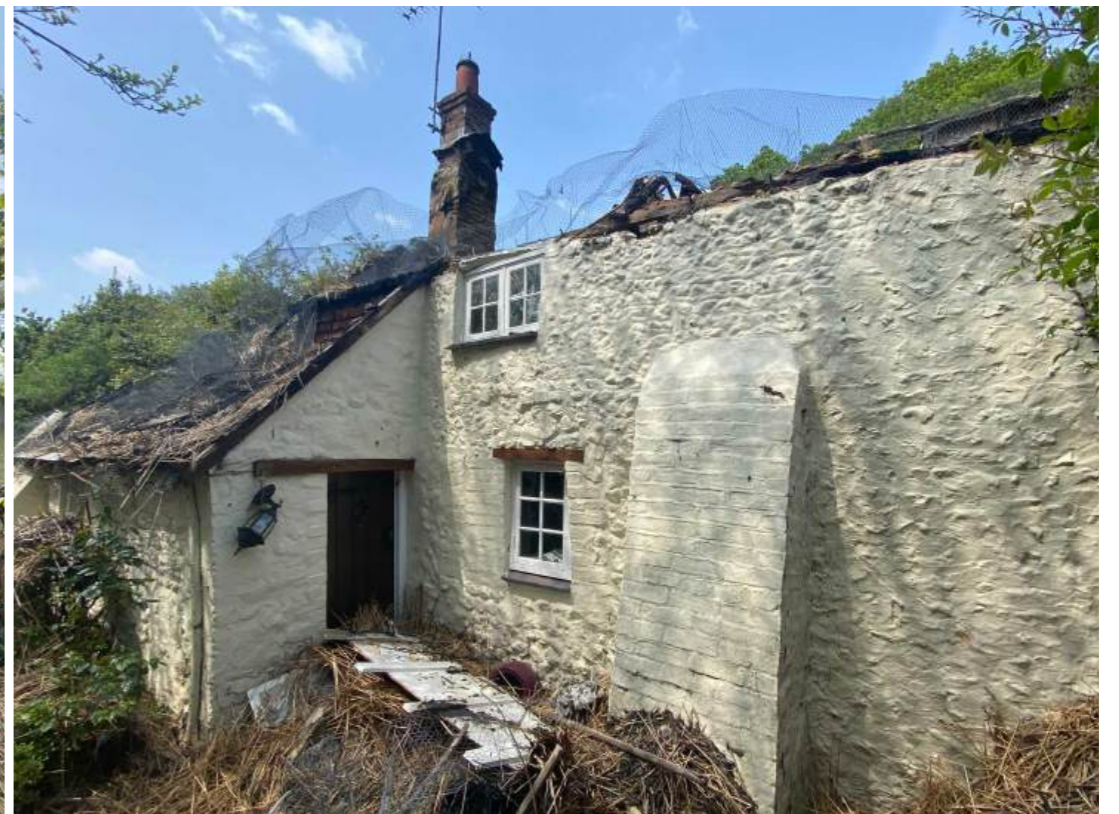
To the rear looking northwest, summer 2023.
