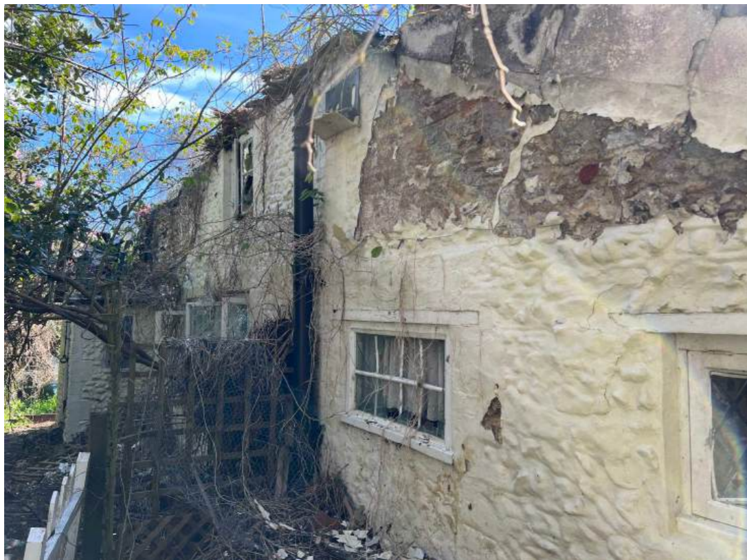
Front elevation from northwest, spring 2025
