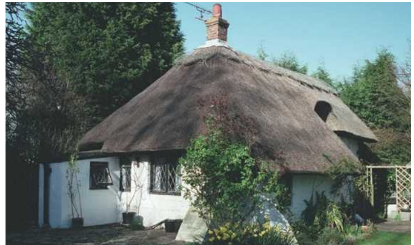
The building in 2003, viewed from the southwest (Mr Robin Earl. Source: Historic England Archive, 2025)
