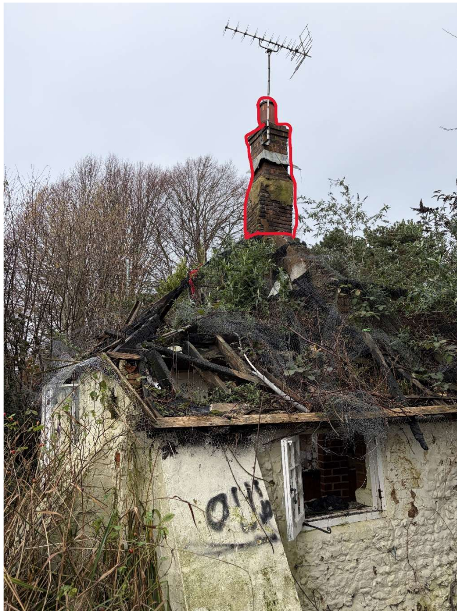
Figure 1. South gable chimney – extent to be dismantled
