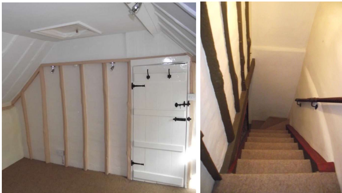
Figure 7 and 8 Record photographs of partition wall to stairwell and bedroom 1.
