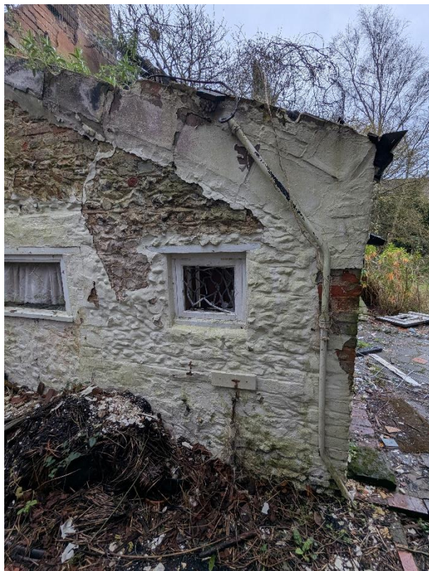
Photo 8 - External wall condition 5
