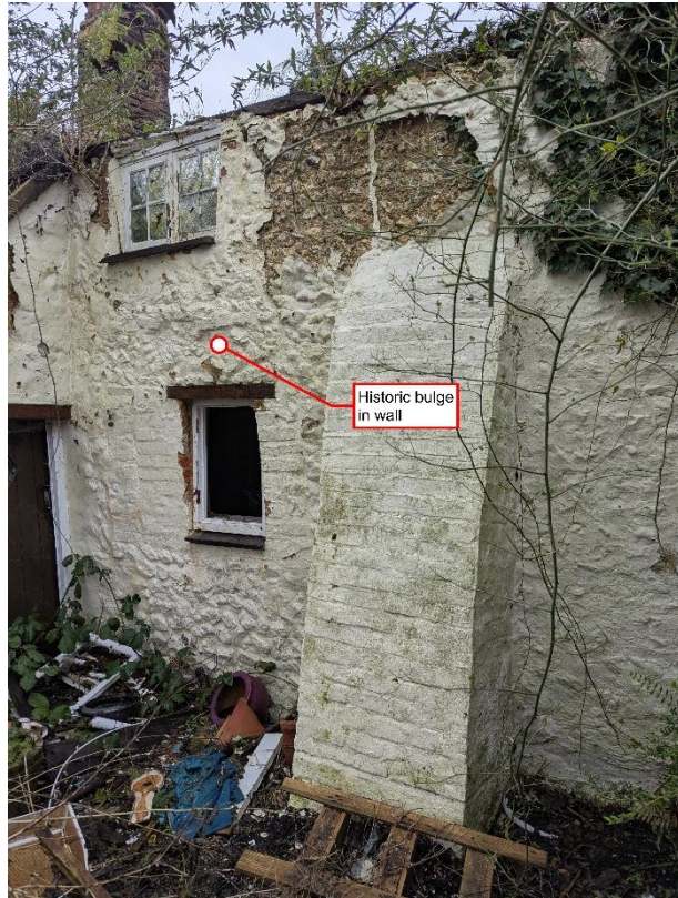
Photo 5 - External wall condition 2
