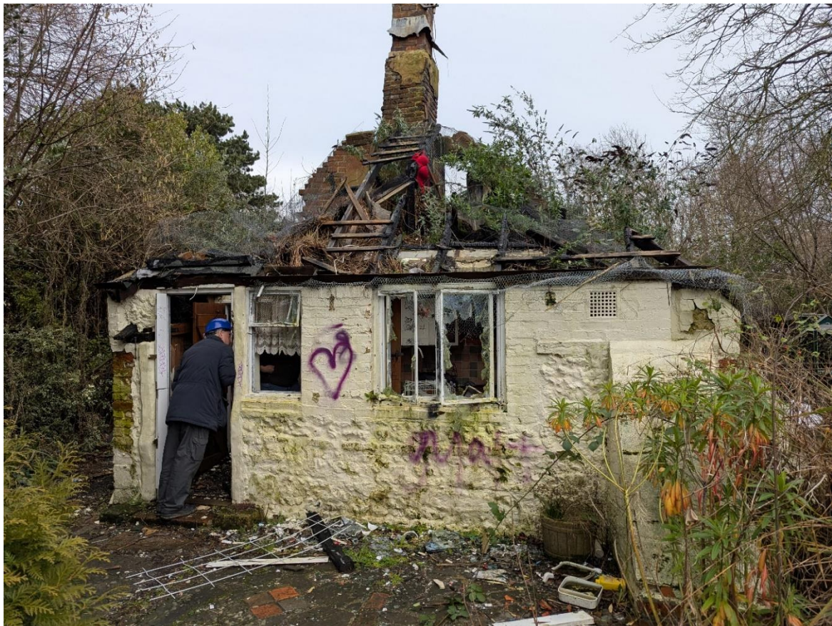
Photo 6 – External wall condition 3
