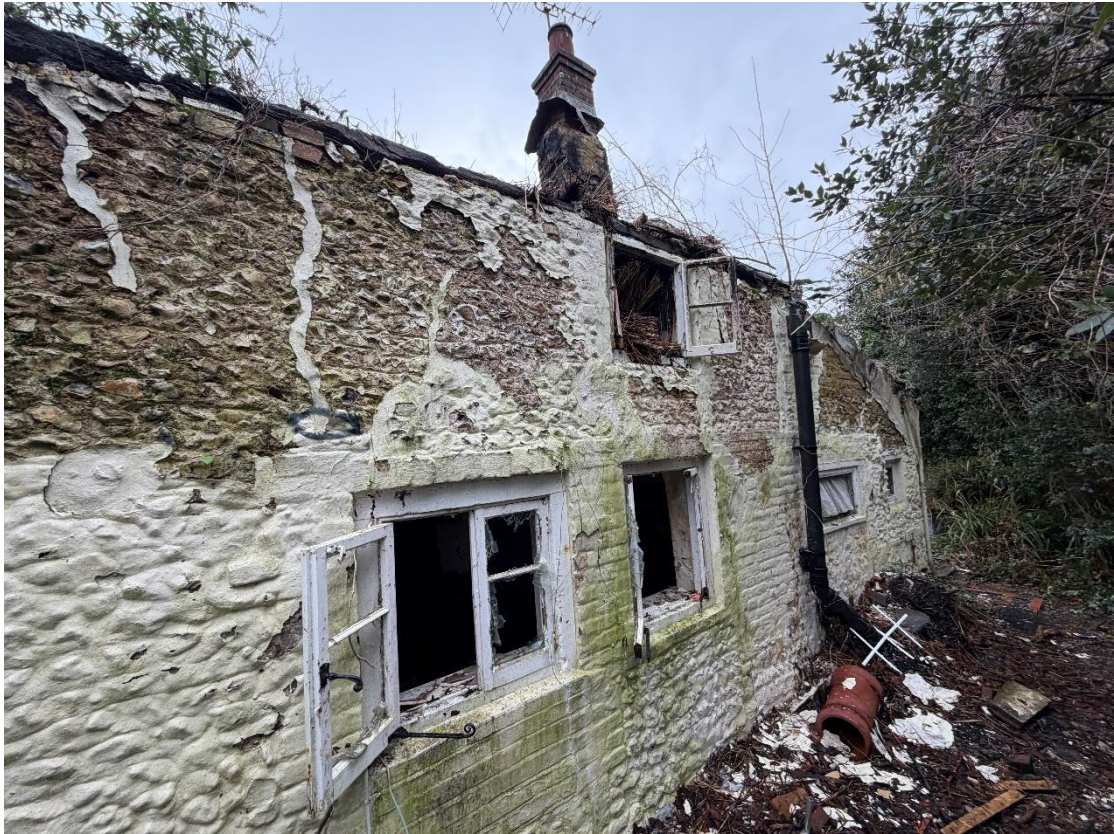
Photo 9 - External wall condition 6
