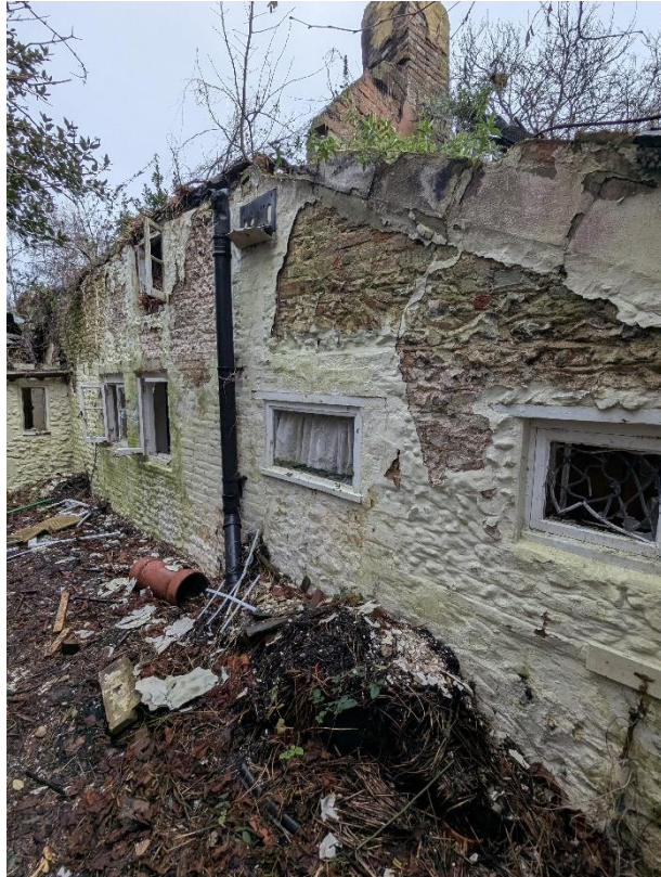
Photo 7 - External wall condition 4
