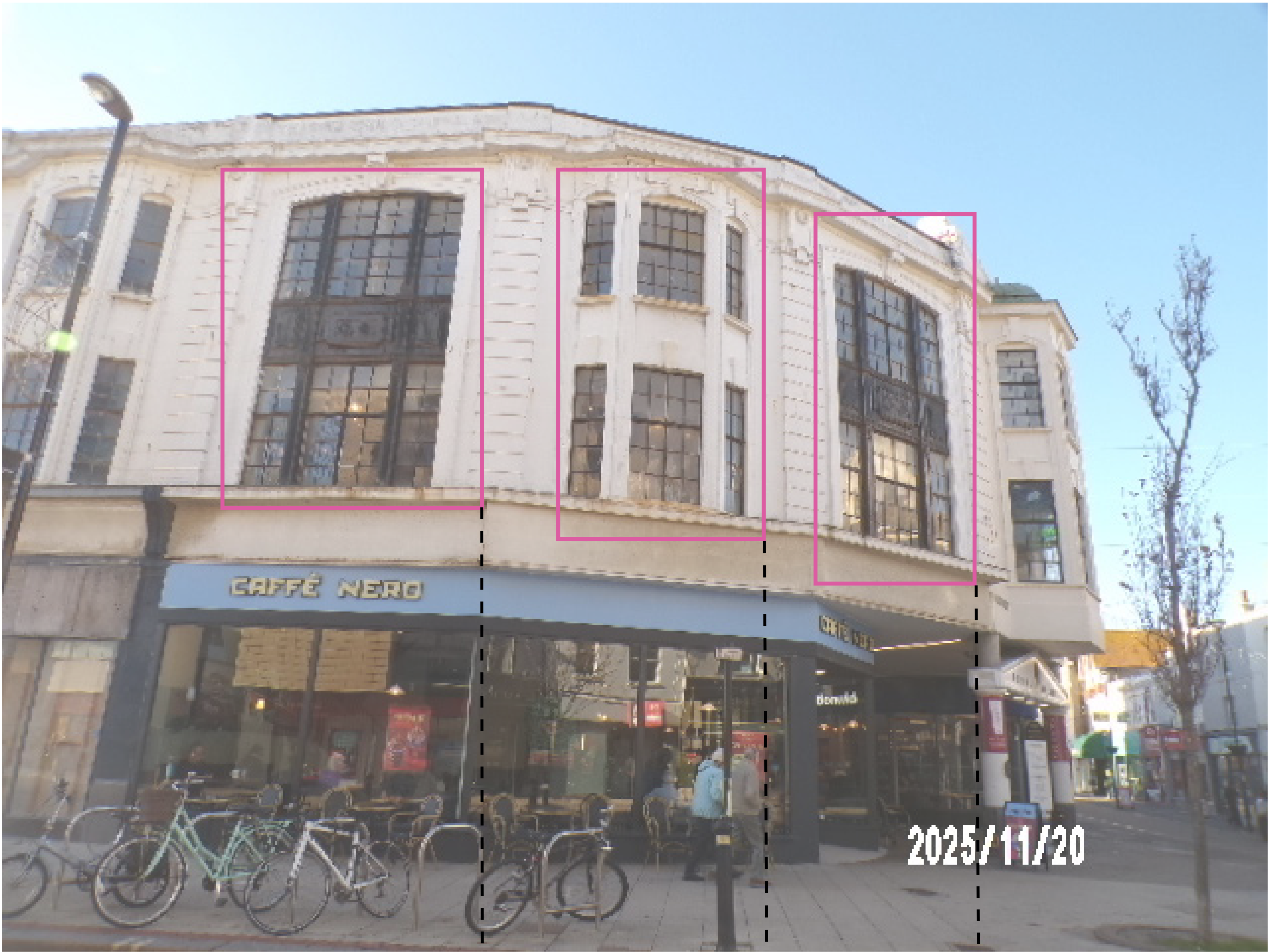
GLAZING EAST FIRST FLOOR - CUSTOMER SEATING AREA SECOND FLOOR - VACANT PARTS
