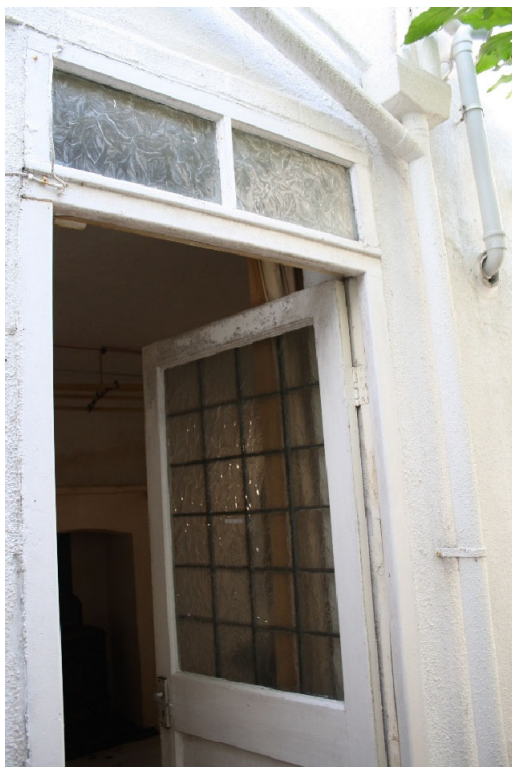
Ground floor D2 & W3 adjacent – both to be overhauled. Non original.
