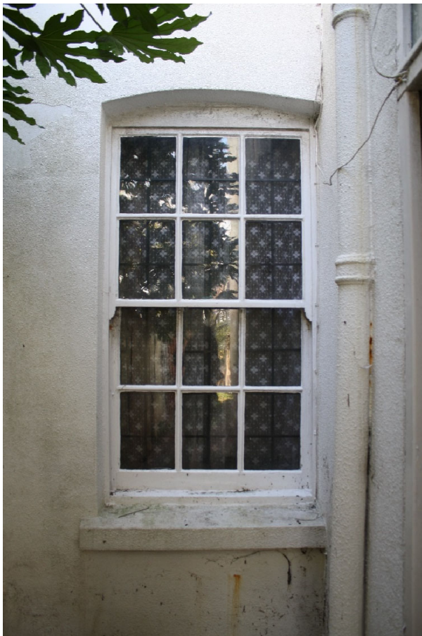
Ground floor W2 – to be overhauled
