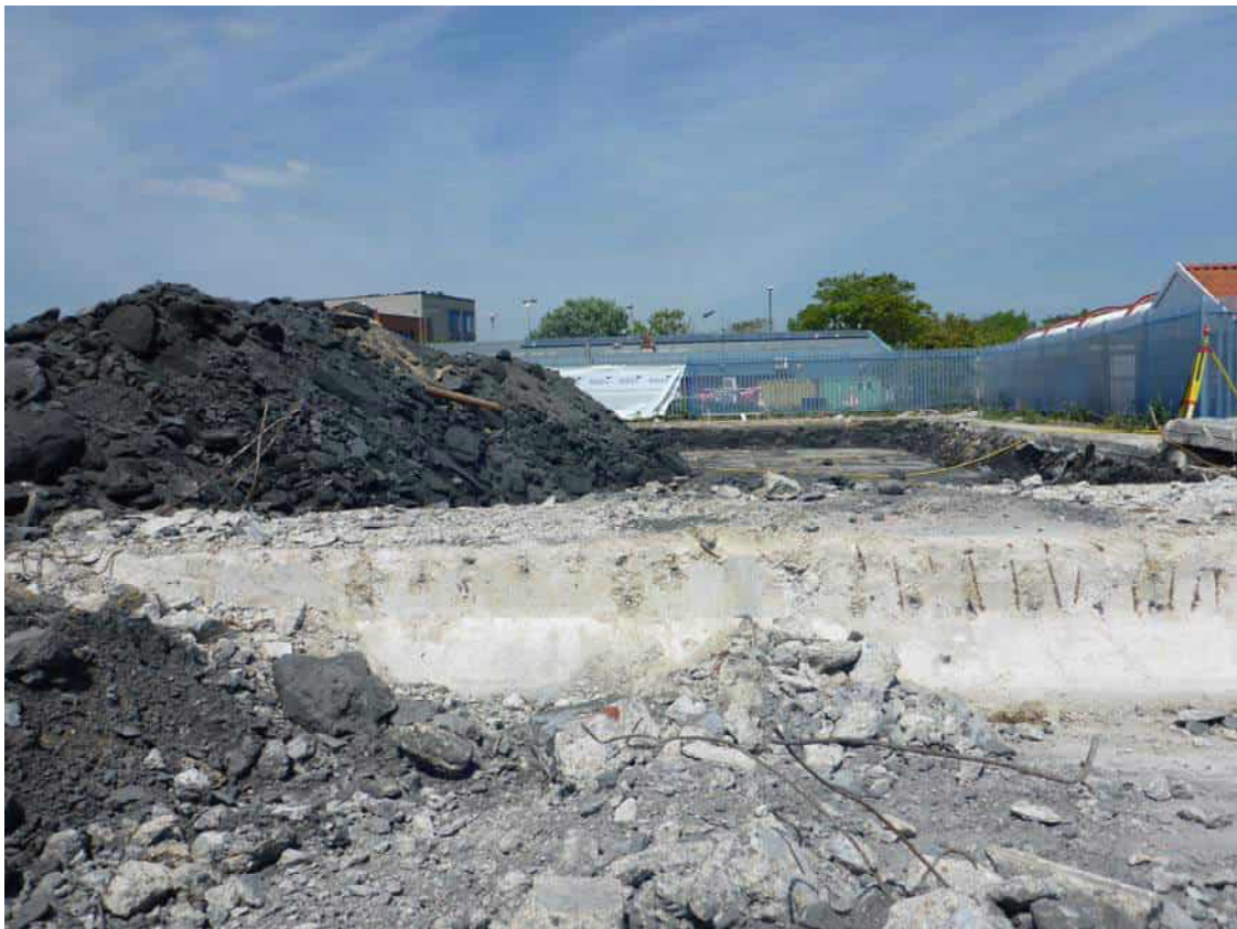
View of PFA (Pulverised Fuel Ash) type material recovered and stored.
