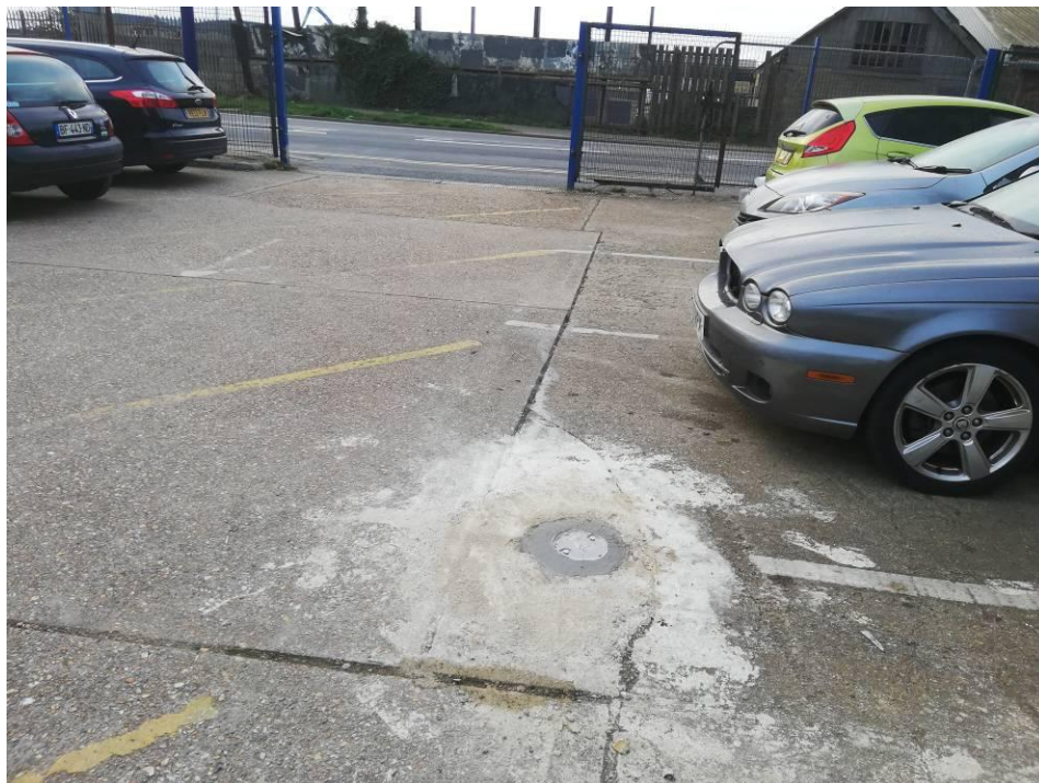
WS4 MONITORING WELL PROTECTED BY FLUSH COVER
