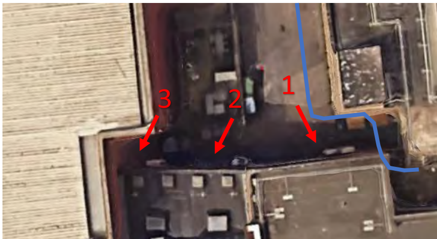
Figure 5. Rear of 60-64 Montague Street Plant Locations (Google Imagery 2023, The Geoinformation Group)
