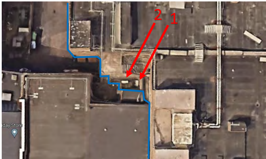
Figure 4. Western Plant Location (Google Imagery 2023, The Geoinformation Group)
