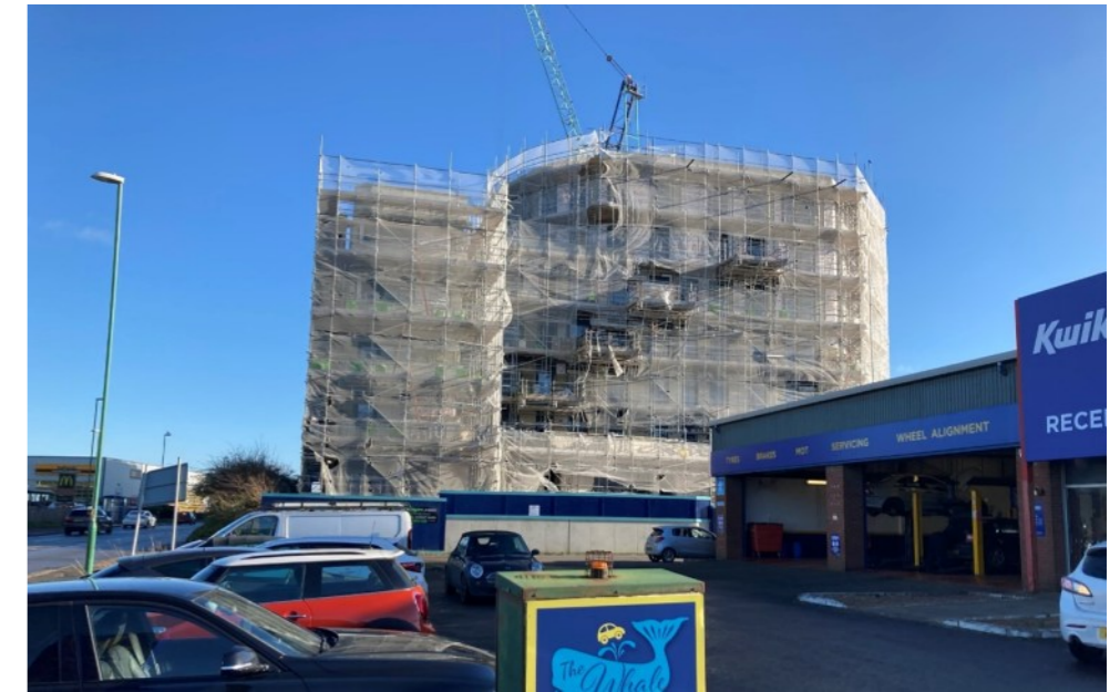
View across the Kwik Fit forecourt onto east boundary
