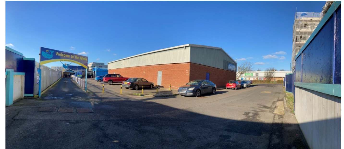
Access to Car Wash facility along the southern boundary
