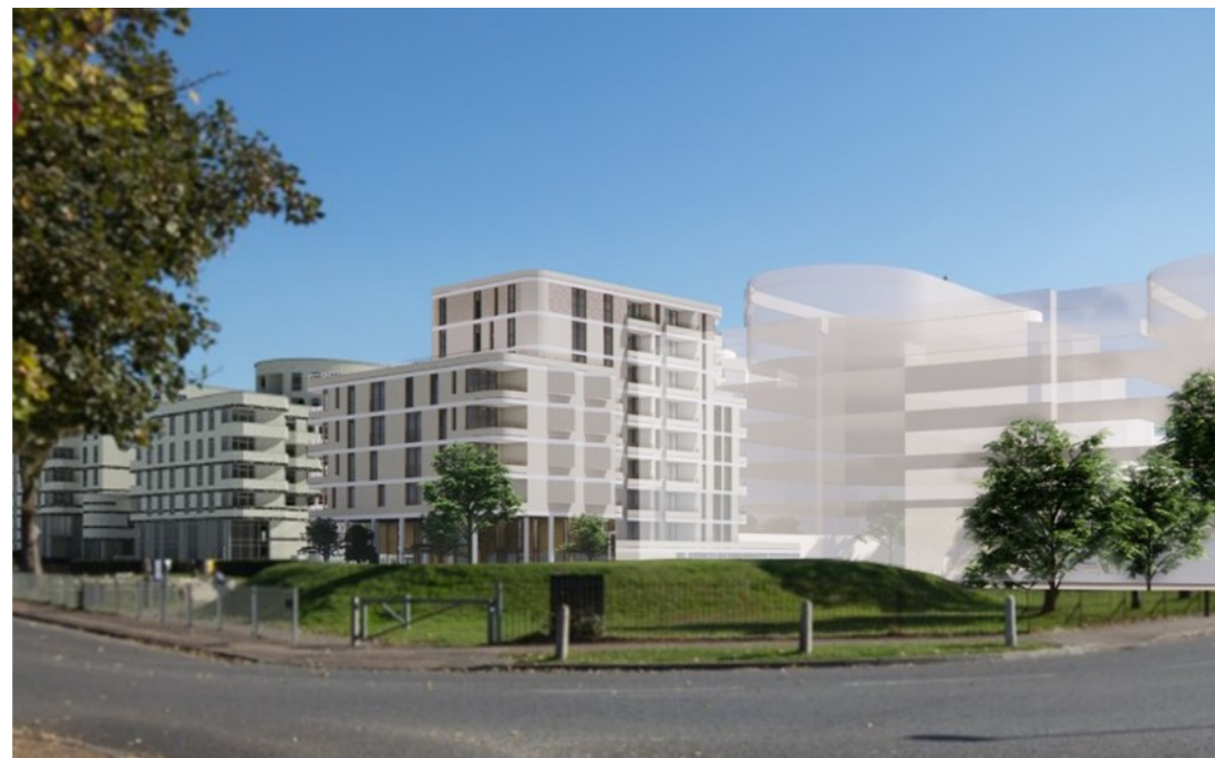
Original design with brick parapet from a distance
