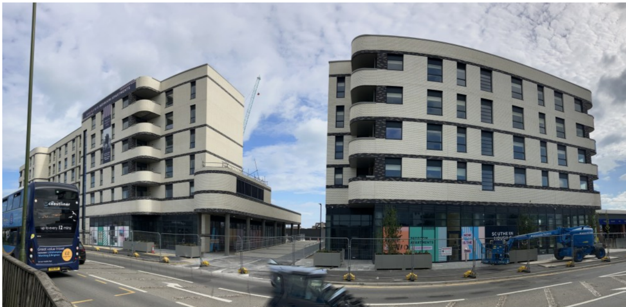
Free Wharf Blocks G1, G2 and H to east from the Proposed Scheme. Ground Floor "base".
