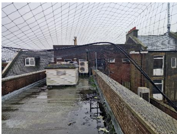
19. Upper flat roof – Roof 2
