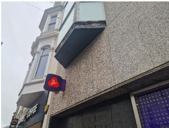
3. Granite cladding to front elevation
