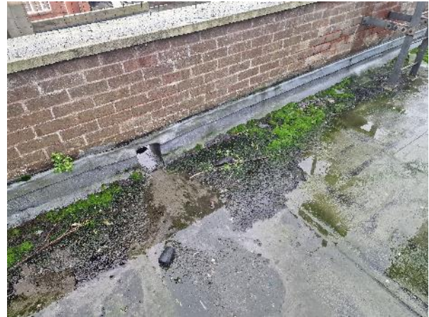
16. Upper flat roof – Roof 2
