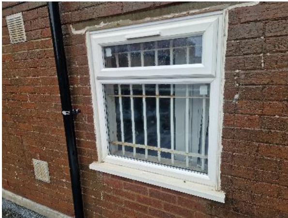
21. Replacement PVCu framed window to rear
