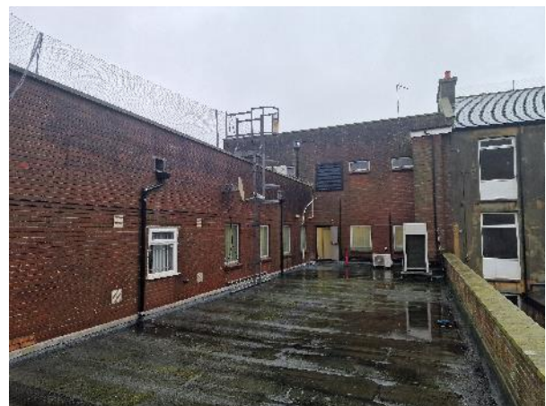
14. Lower flat roof to rear
