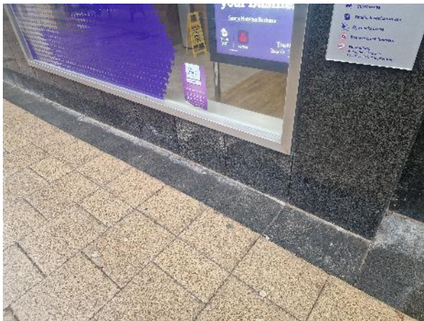
7. Granite to shop front
