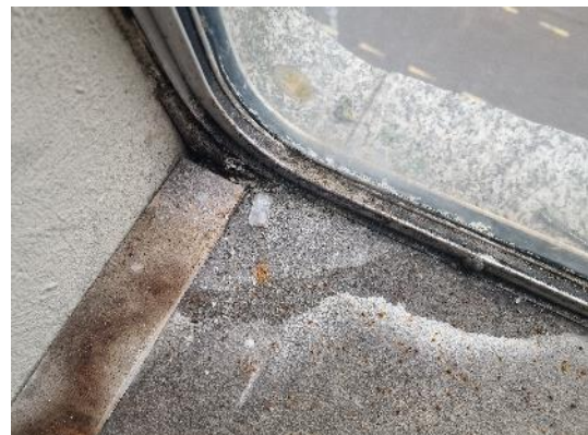
Photograph F – Typical window to front elevation
