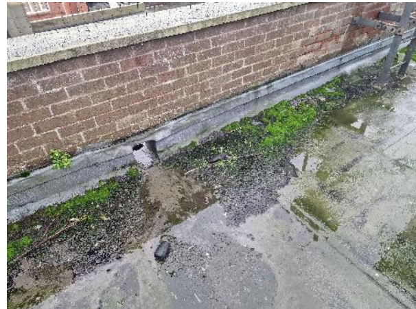
16. Upper flat roof – Roof 2
