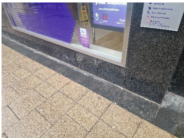
7. Granite to shop front
