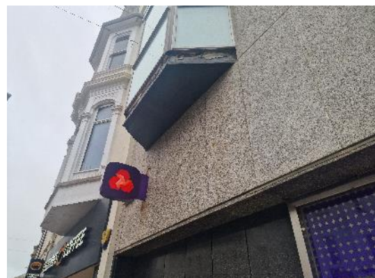
Photograph D - Cladding
