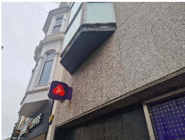
3. Granite cladding to front elevation
