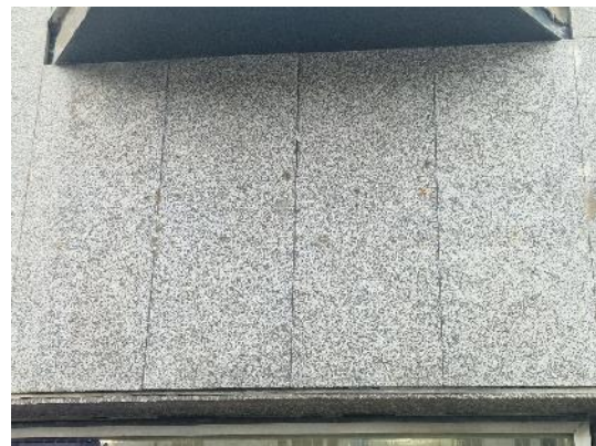
Photograph C – Granite cladding to front elevation
