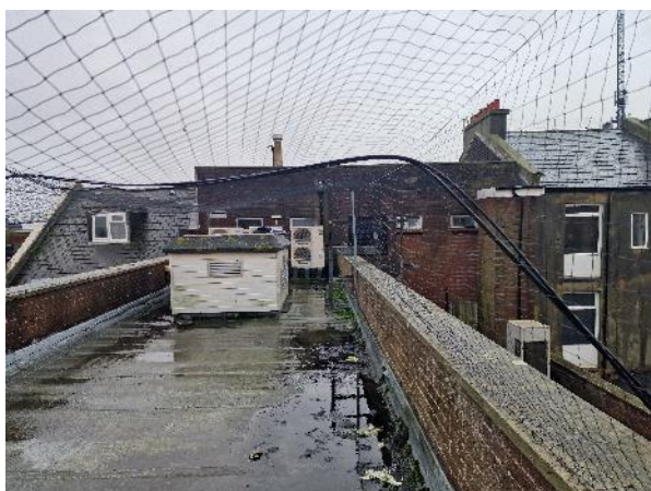
19. Upper flat roof – Roof 2
