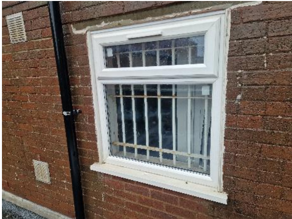
21. Replacement PVCu framed window to rear
