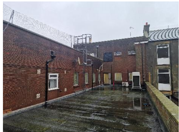
14. Lower flat roof to rear
