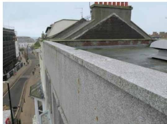
Photograph A – Coping stones to main roof
