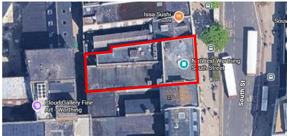
Site aerial photograph
