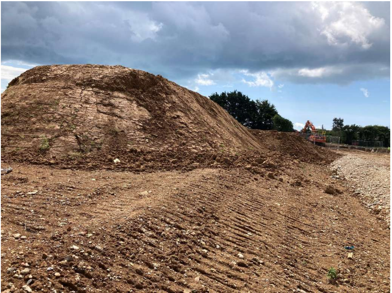
Figure 4: Billingshurst soil stockpile SL04/05
