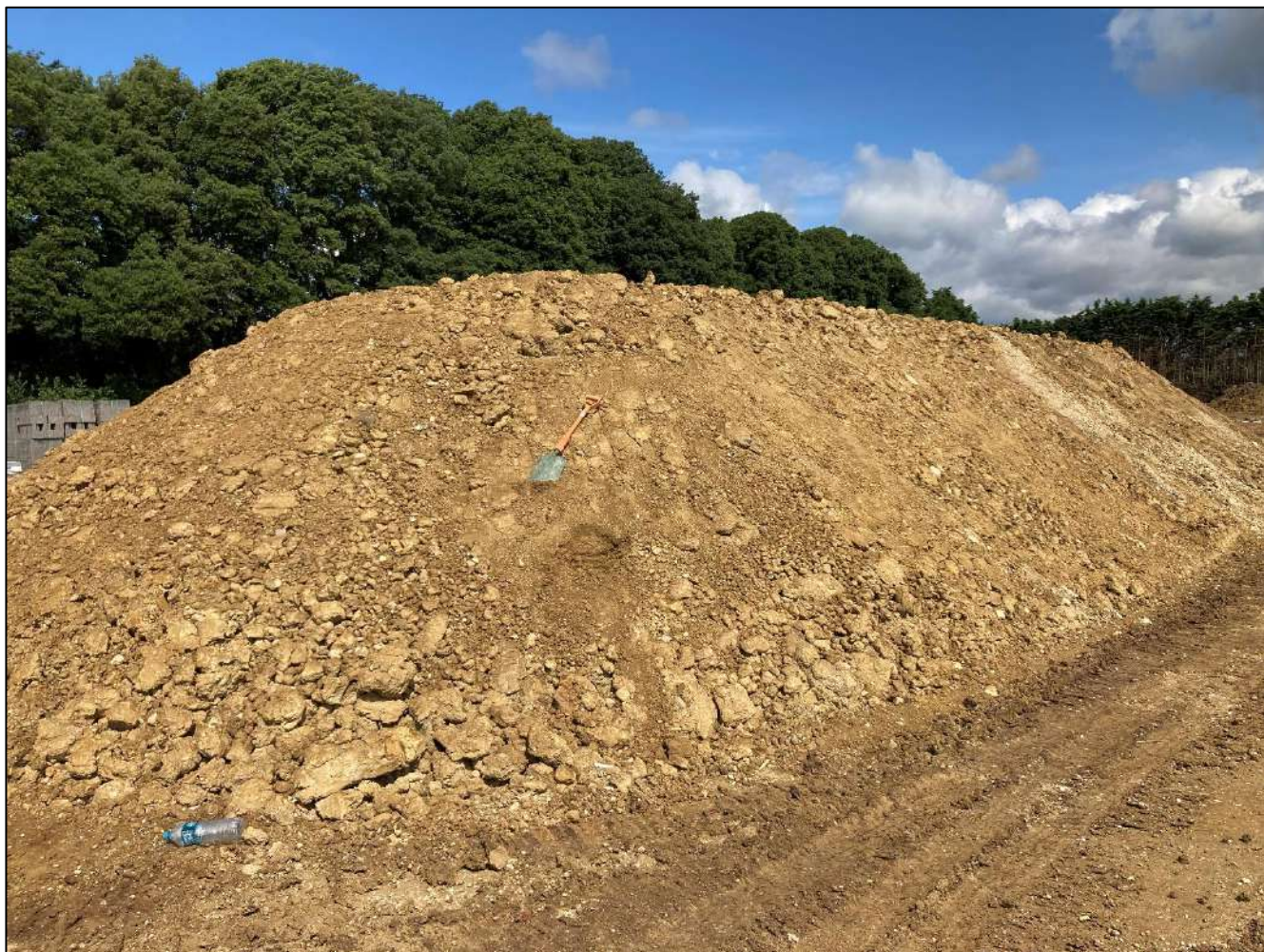
Figure 2: Billingshurst soil stockpile SL02
