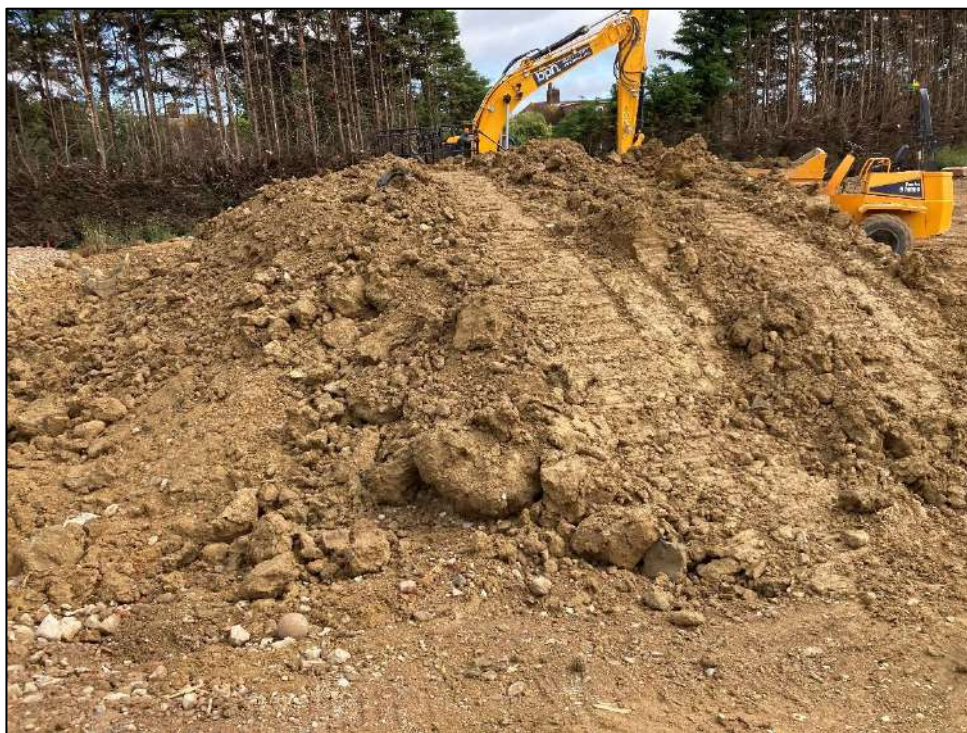
Figure 1: Billingshurst soil stockpile SL01
