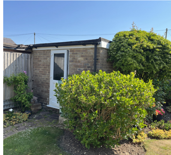
Rear of garage
