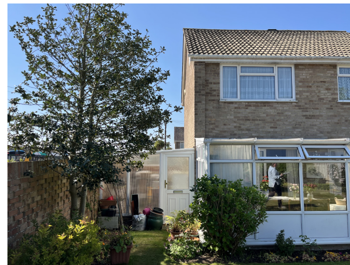
Rear garden - looking west towards the rear gardens of No.s 4 and 6
