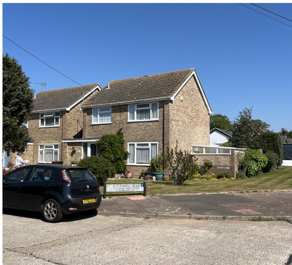
Front façade - facing Cherwell Road
