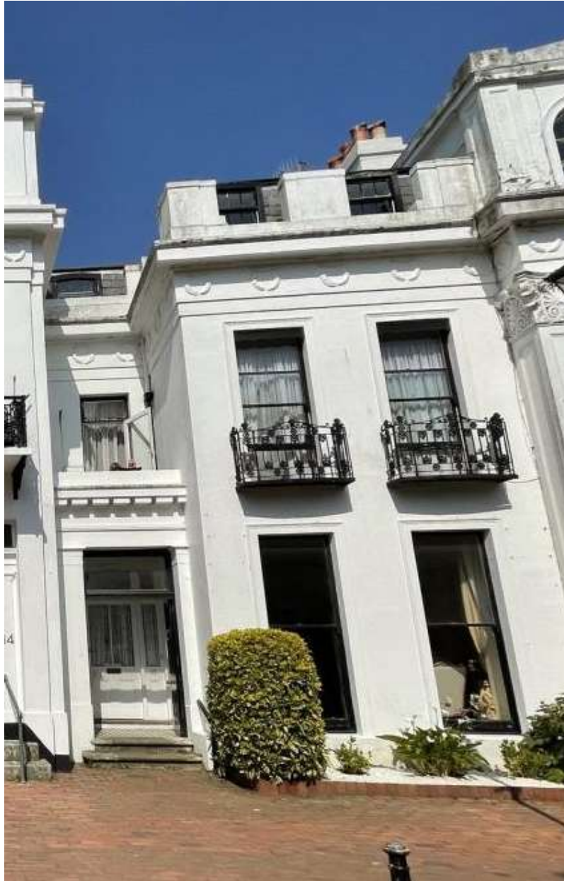
Fig 1. Front elevation to 13 Park Crescent, Worthing.
