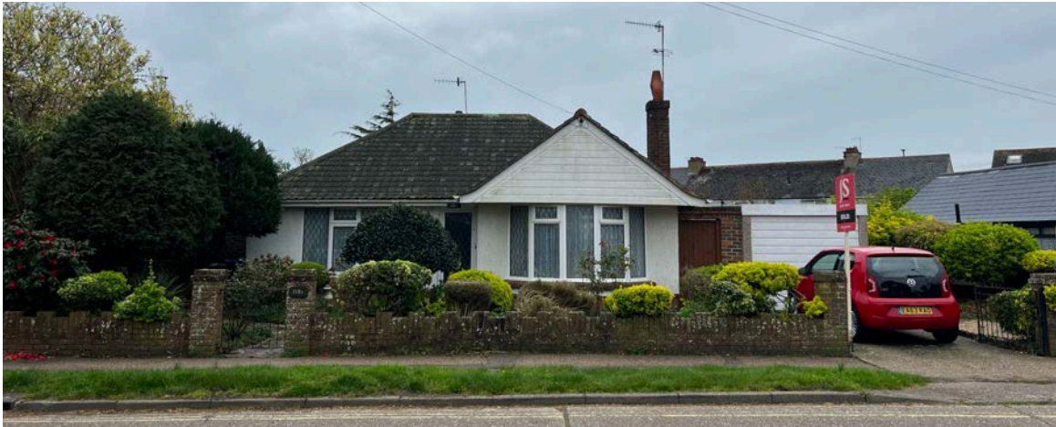
Figure 04. Photo of the existing site & structure (facing south)
