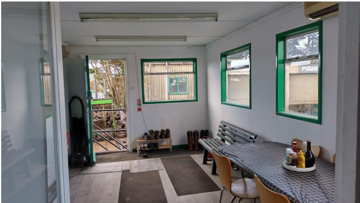
Figure 4: The utility / dining room, looking towards the entrance door off the metal stairs
