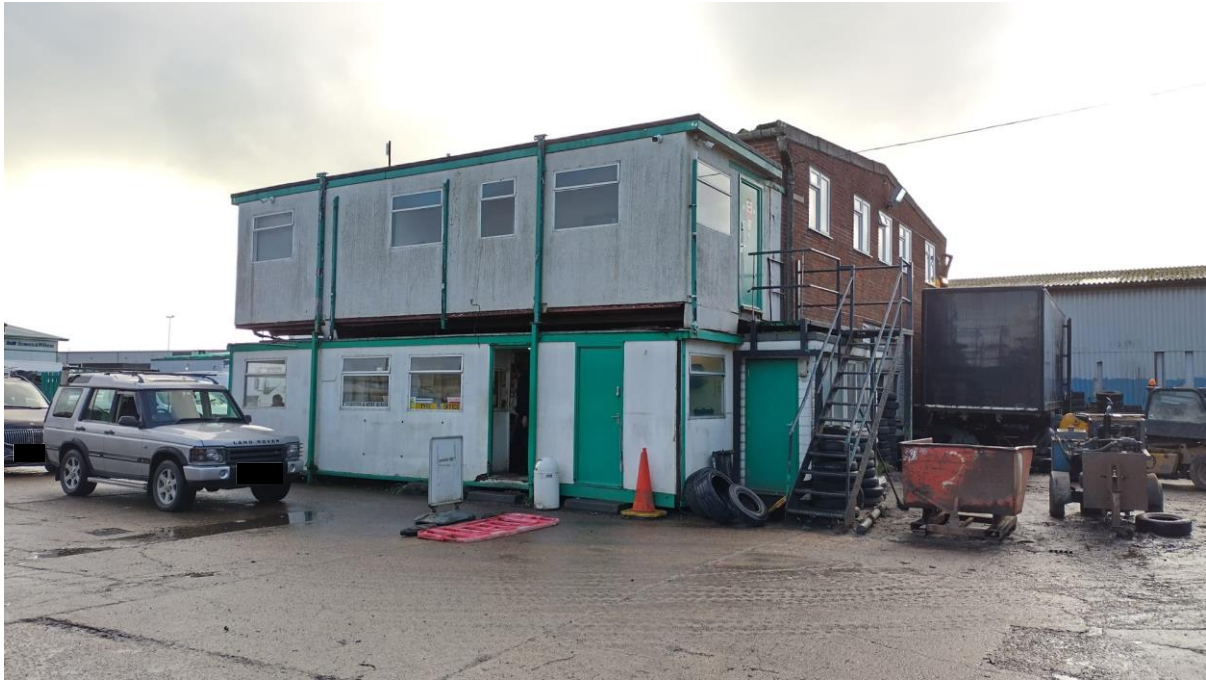
Figure 1: North elevation, with external metal stairs leading to first floor accommodation
