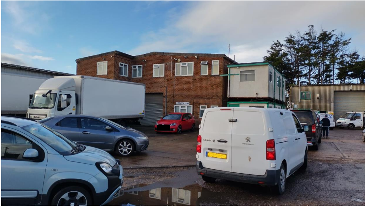
Figure 3: East elevation, facing Dale Road
