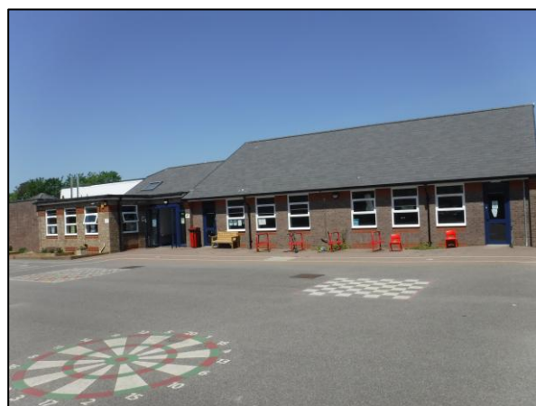
Plate 3: School looking northwest
