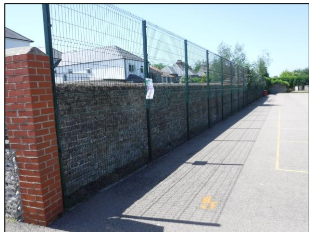
Plate 8: Brick wall looking west
