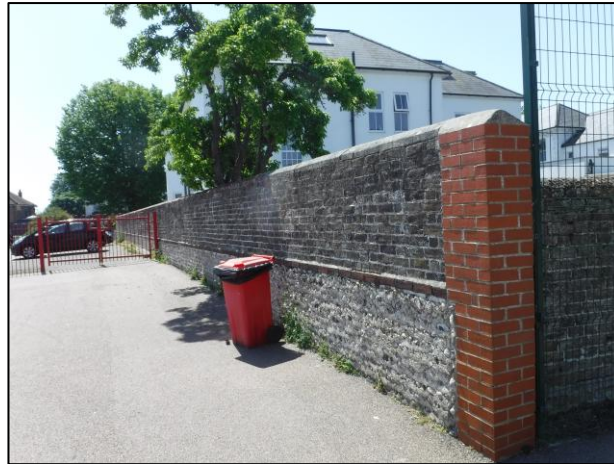
Plate 9: Brick and flint wall looking southwest
