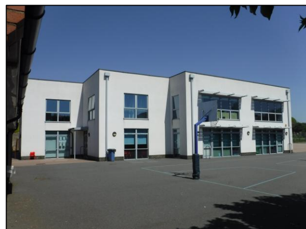
Plate 4: Classroom block looking north
