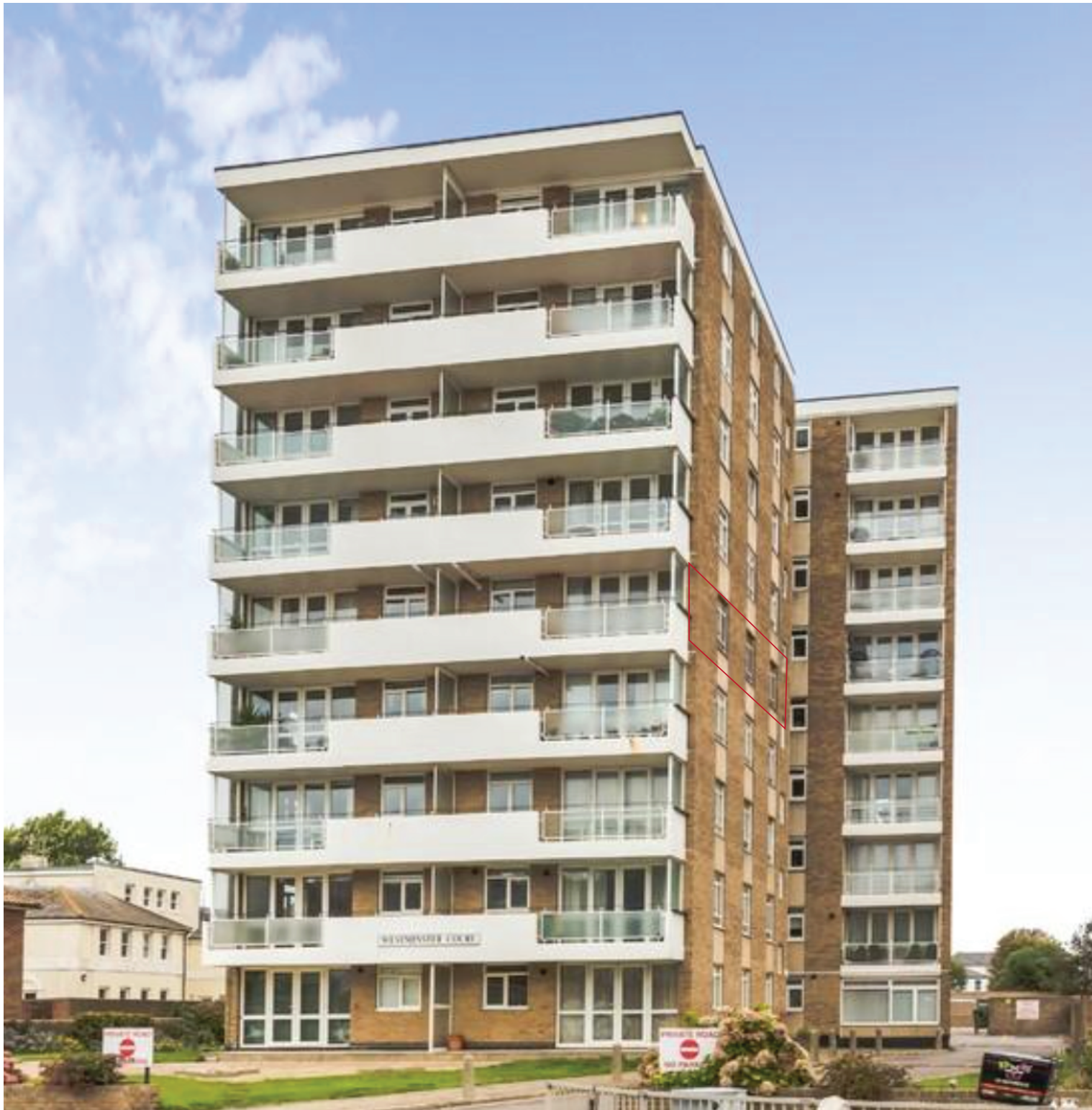
1. BEDROOM 1 REPLACEMENT WINDOW
