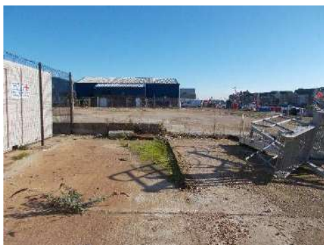
Concrete surfacing with drains in the eastern area of the site
