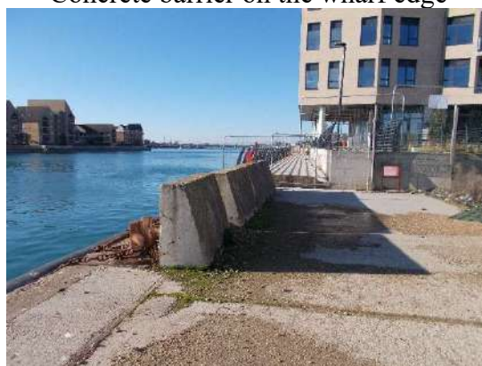
Concrete barrier on the wharf edge
