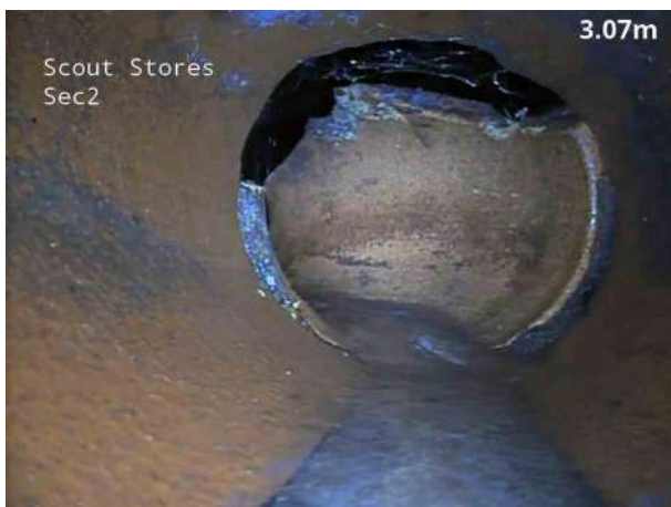
5, 00:00:41, 3.30 m Finish node, manhole, reference: 7601
