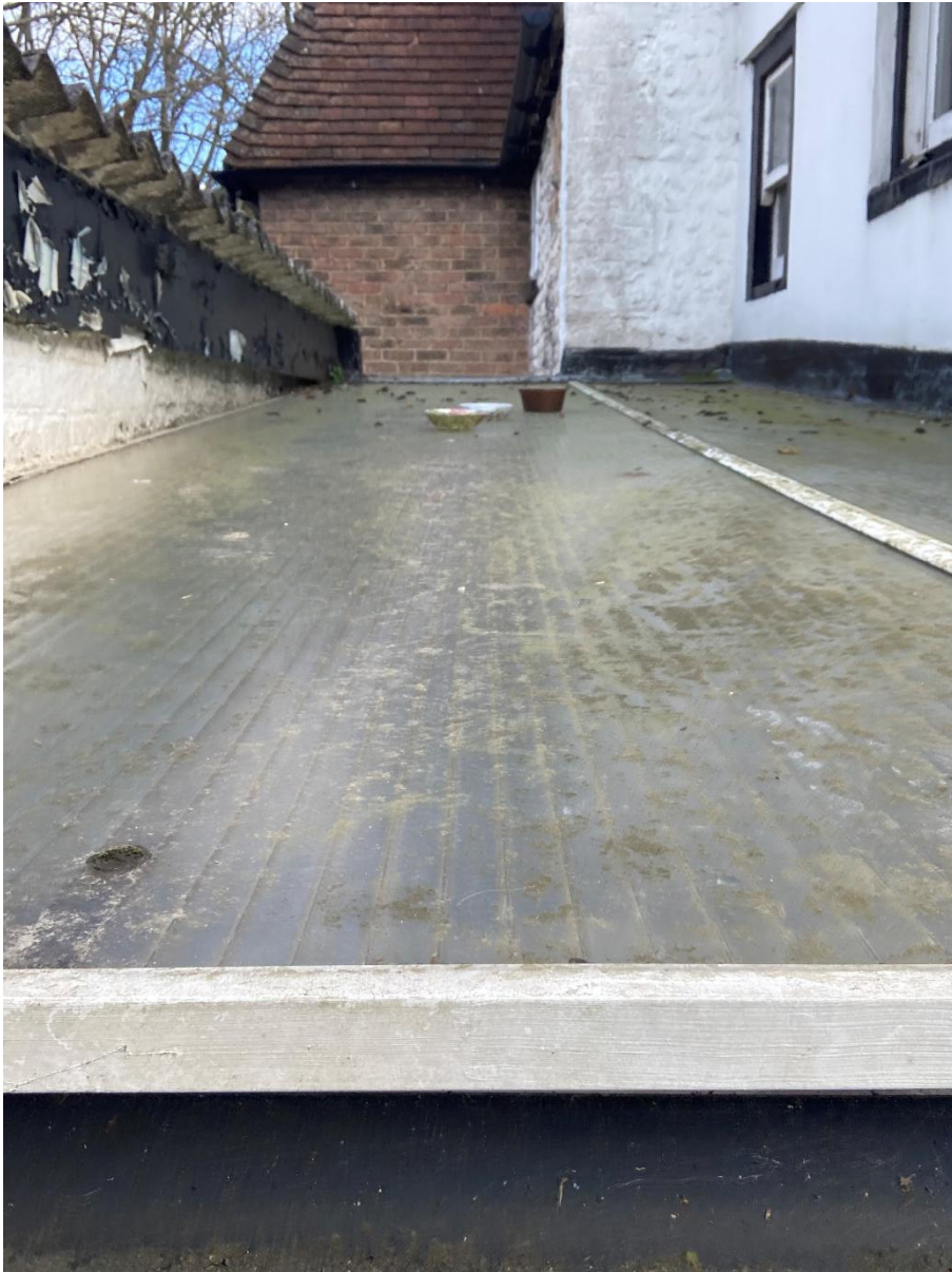
Image 10 – Polycarbonate roof viewed from outside
