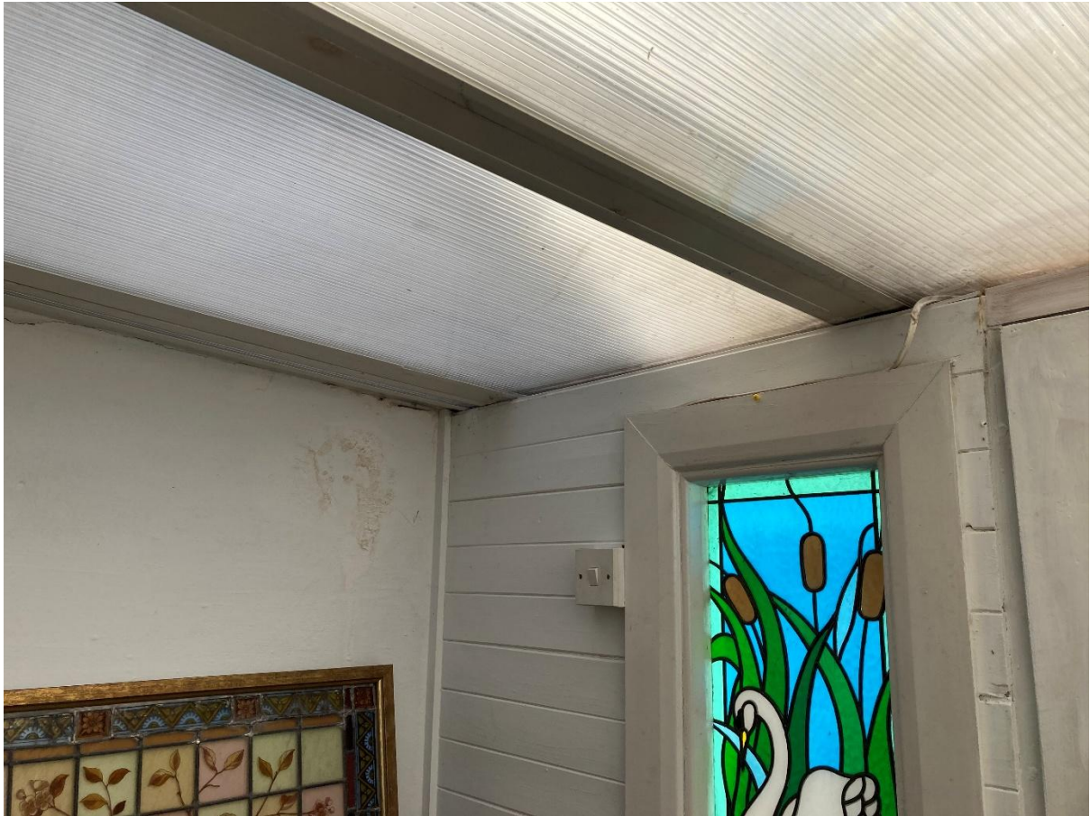
Image 09 – Polycarbonate roof & part of stained glass window viewed from inside
