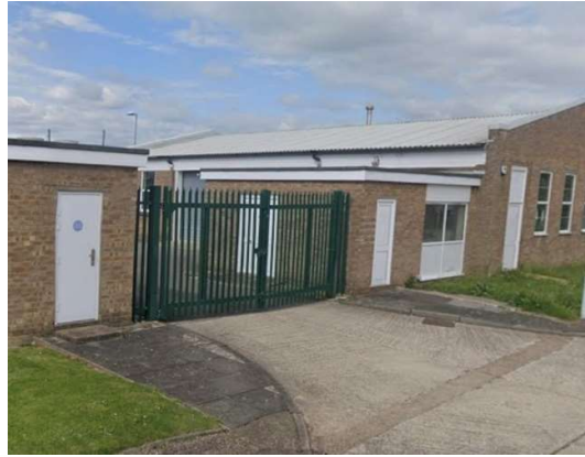
Shared Access to Units 5 & 6
