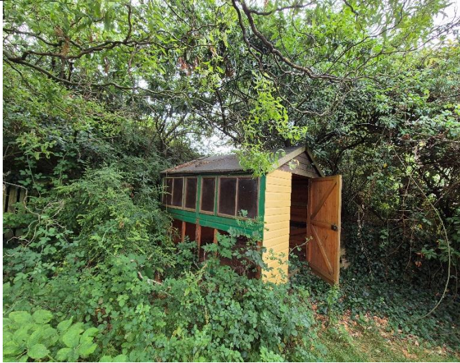
Photo 5: Shed on Site
