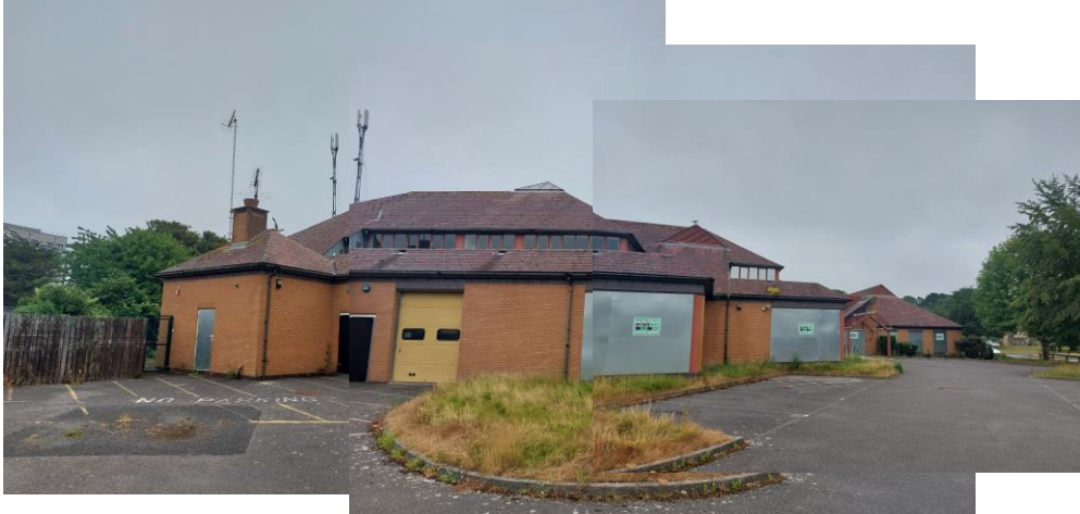
Image 01 – View looking east of the existing Building B1 and other neutral grassland swards found on the western aspect of the site.
