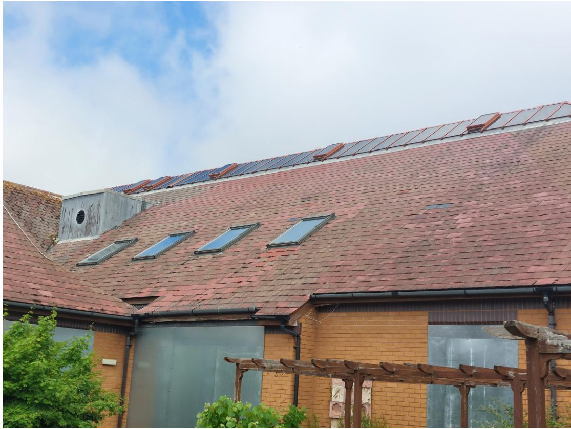
Image 05 – View of the western aspect of Building B1.
