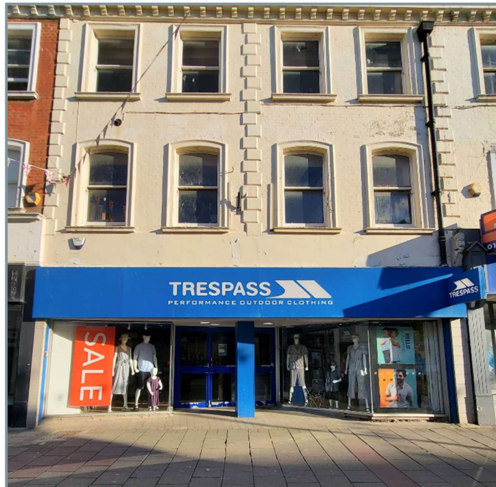
Above: The site
